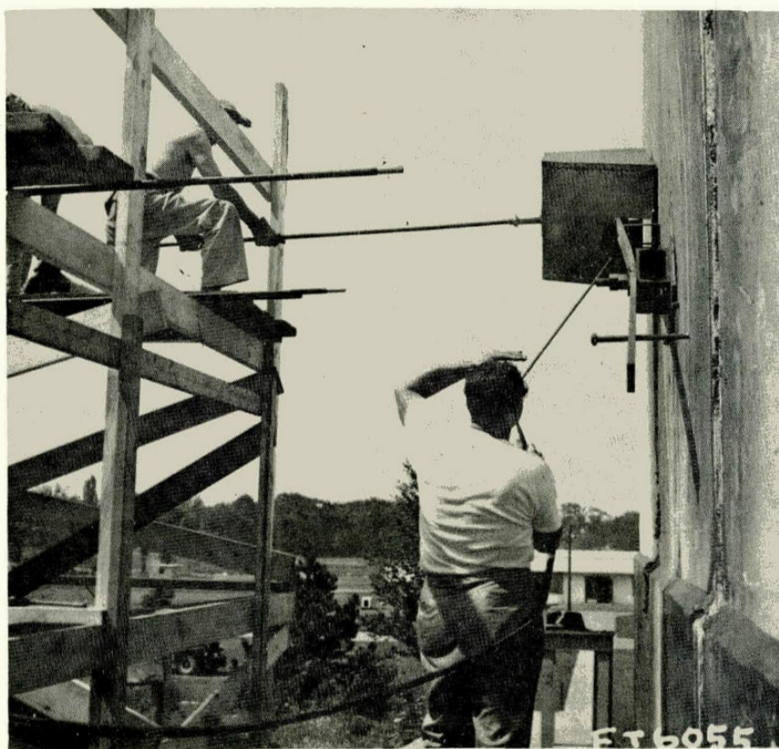
FIG. 1 FIRST STEP: HEATING THE LANCE TIP TO MELTING POINT
