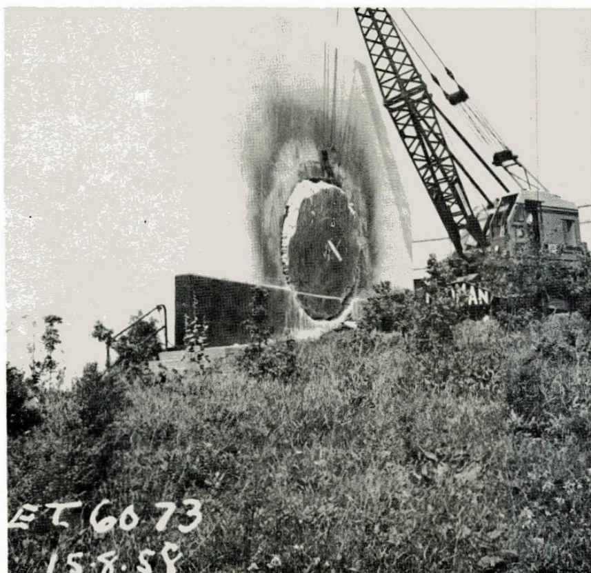
FIG. 6 25-TON CRANE TAKES THE LOAD.
