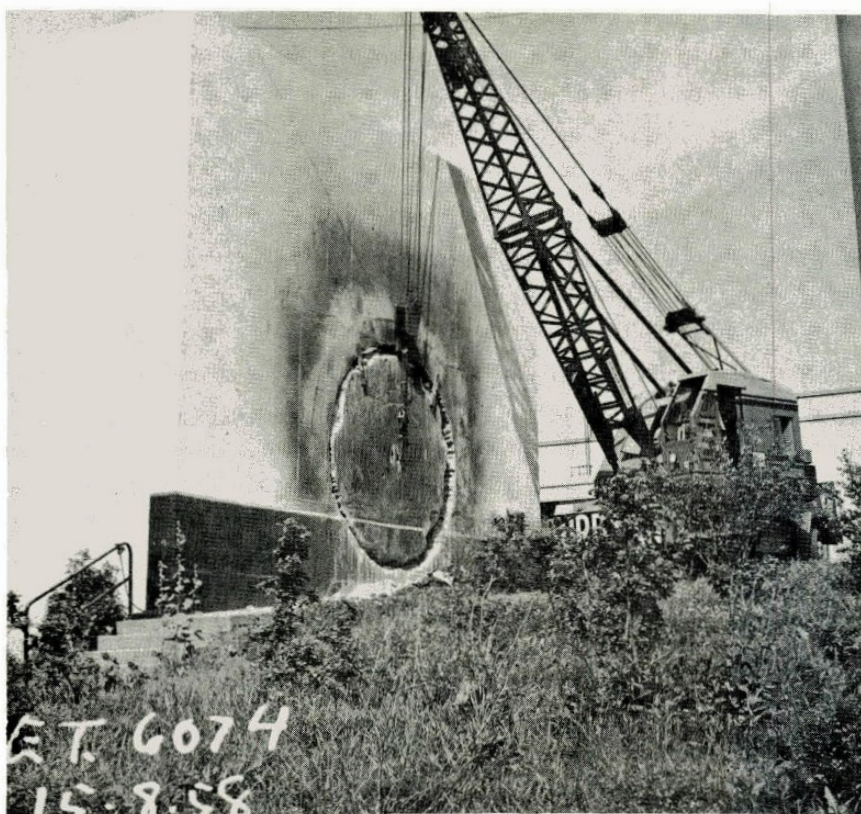
FIG. 5 REMOVAL OF CONCRETE DISC.
