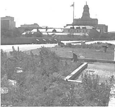
Garden roof system on Toronto City Hall
