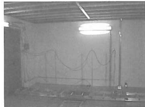
One of the test rooms in IRC's new world-leading flanking research facility
