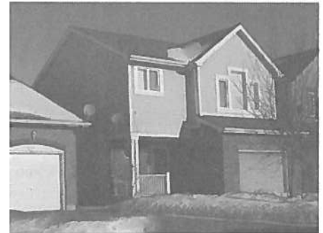
The 2005 NBC has incorporated a new climate indicator called the moisture index to help address the issue of protection of housing against precipitation
