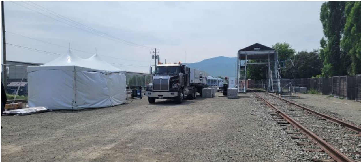
Figure 5: Refuelling and maintenance station
