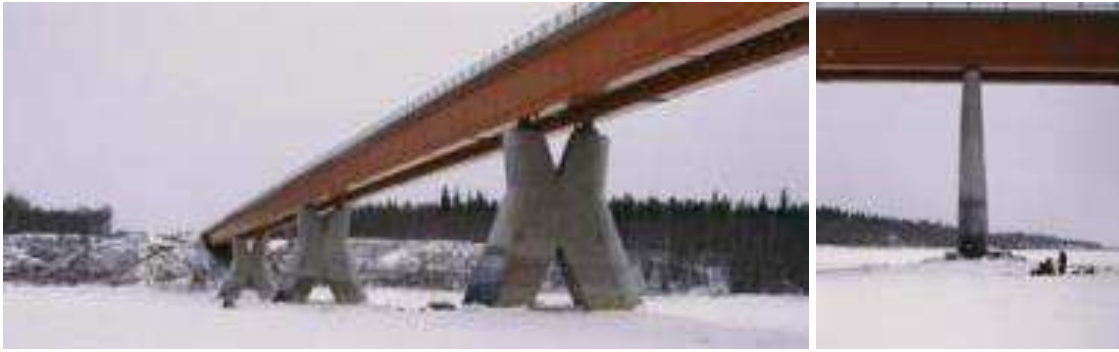
Figure 5. Bridge crossing at Fort Vermillion.
