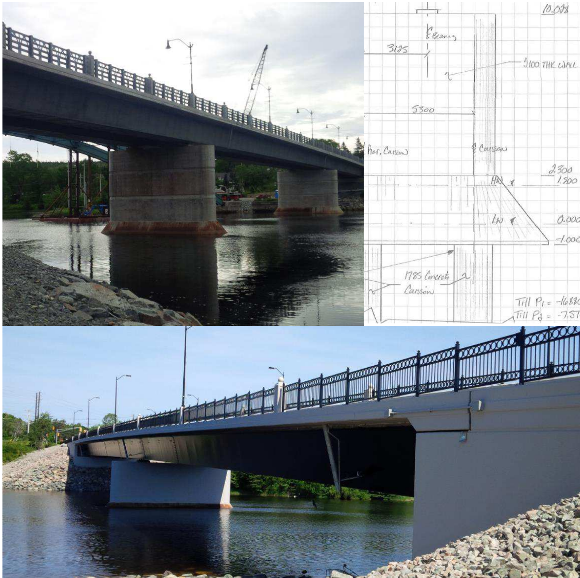
Figure 8. Top left) The East River Bridge, in Sheet Harbour NS - courtesy of NSDTIR. Top right) Schematic of the piers geometry (from a technical memo provided by the NSDTIR). Bottom) The new Sydney River Bridge - courtesy of Transportation and Infrastructure Renewal.
