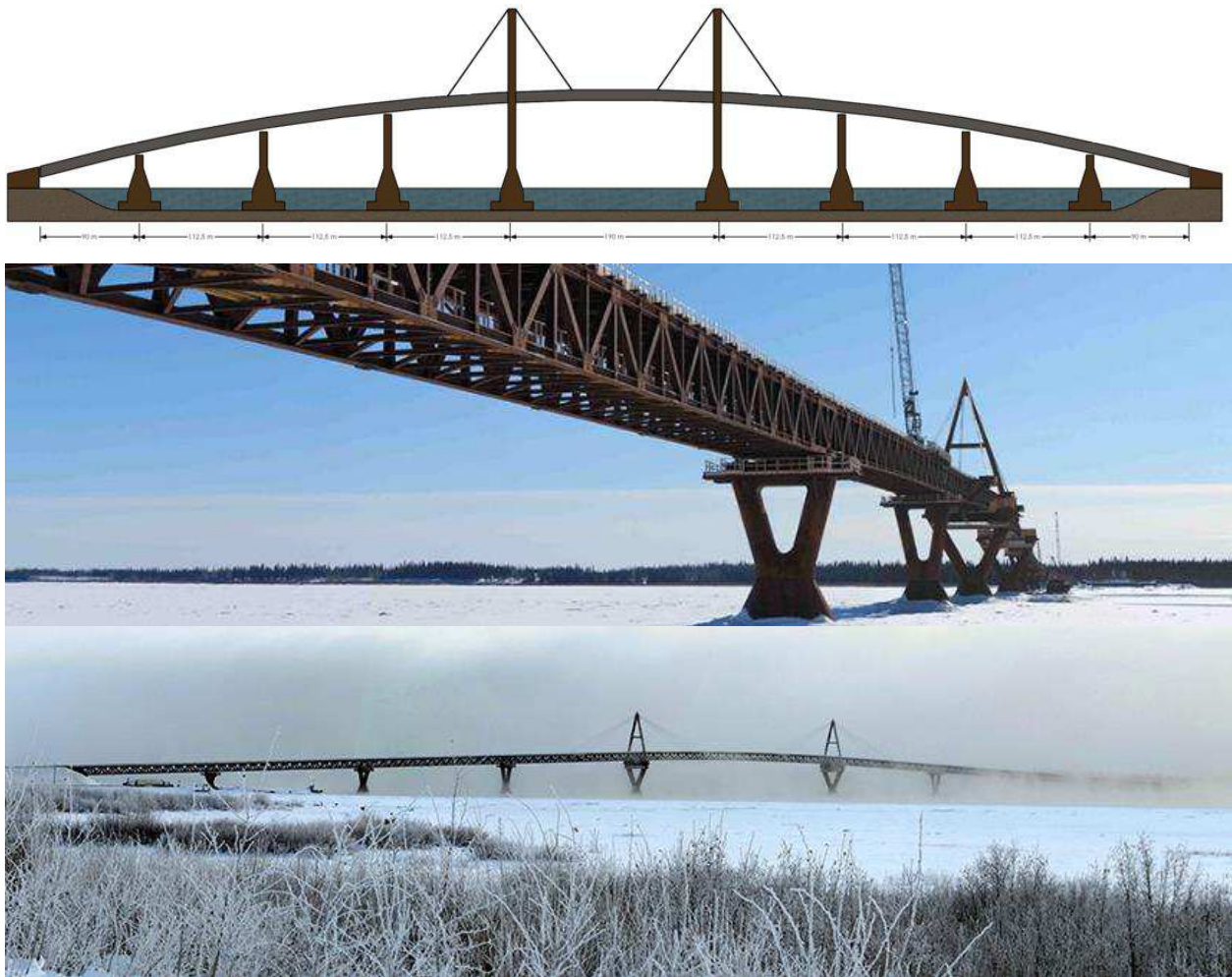
Figure 10. Deh Cho Bridge, crossing the Mackenzie River, in the NWT. Top) Structure drawing (source: Wikimedia 6 ). Middle and bottom) Near and far range views of the bridge (source: The Deh Cho Bridge Project website by NWT Transportation 7 )
