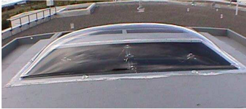
Figure 9 Clear rectangular bubble as installed on the box roof.
