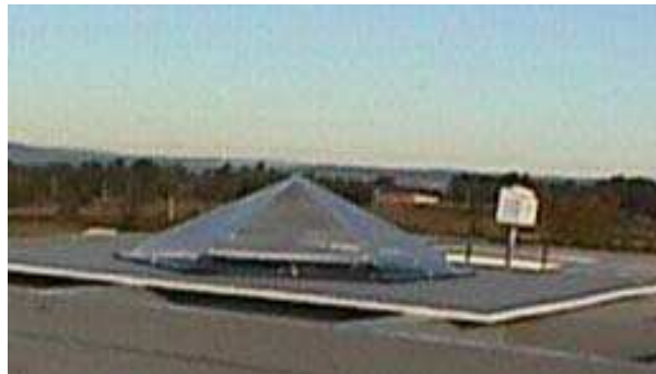
Figure 8 Clear hexagonal pyramid as installed on the box roof.
