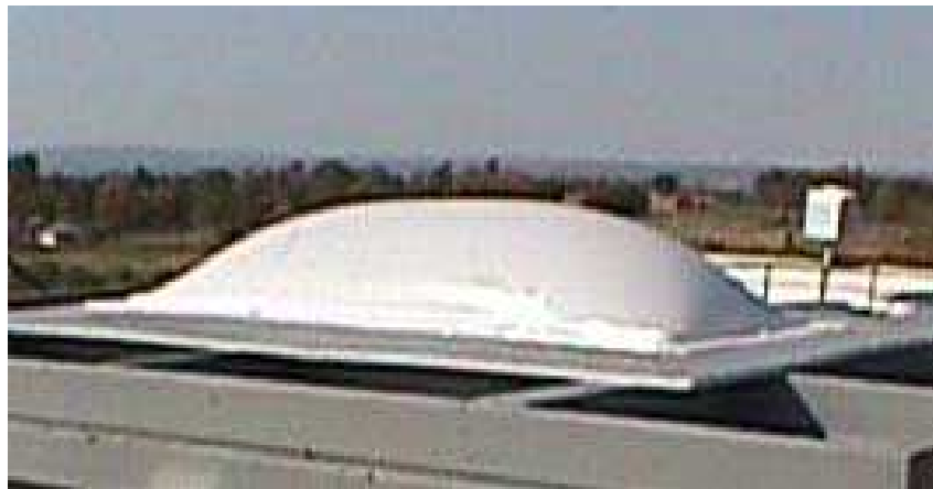
Figure 10 White rectangular bubble as installed on the box roof.
