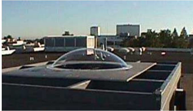
Figure 6 Clear circular dome as installed on the box roof.
