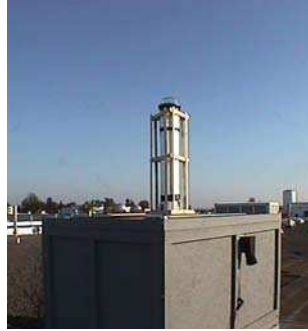
Figure 12 Tubular skylight as installed on the box roof.
