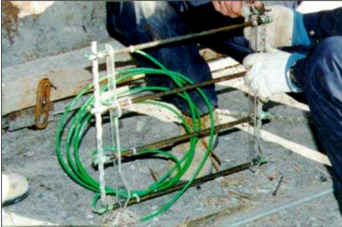
**Figure 4: Special rebar ladder before installation in the parapet form**
