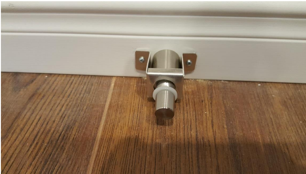
Fig. A. 6. PFS placed on the surface of a baseboard trim (living room, 1st floor).
