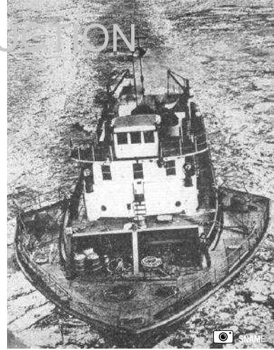
Fig. 5. An ice plow attached to a river tender type Coast Guard Cutter breaking ice on the Mississippi river system (Johnson 1946).
