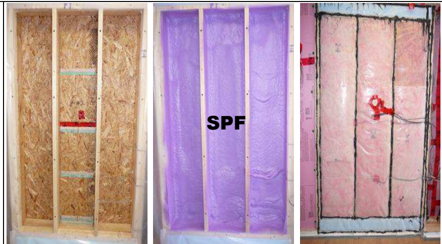
Figure 15. Wall 5 (SPF) - Interior wood frame prior to (i) & following installation SPF insulation in stud cavities (ii), & placement of 178 mm of GF insulation & PE vapour barrier (iii)
