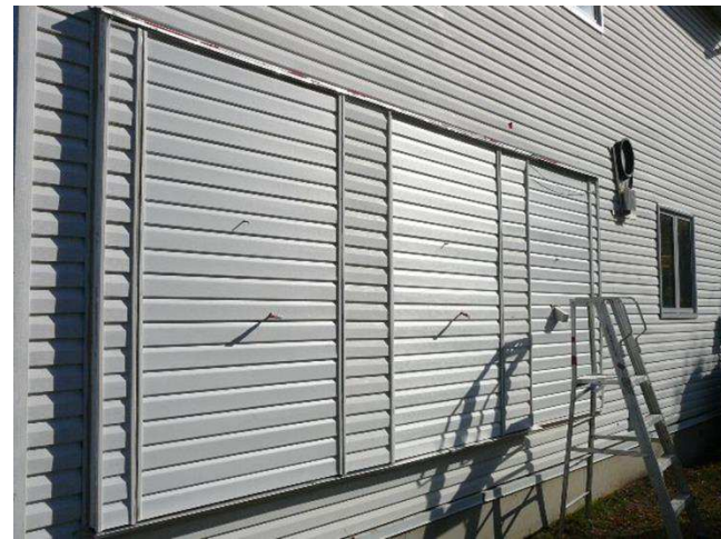
Figure 9. Installation of W1, W2, & W3 in FEWF showing exterior cladding (vinyl siding)
