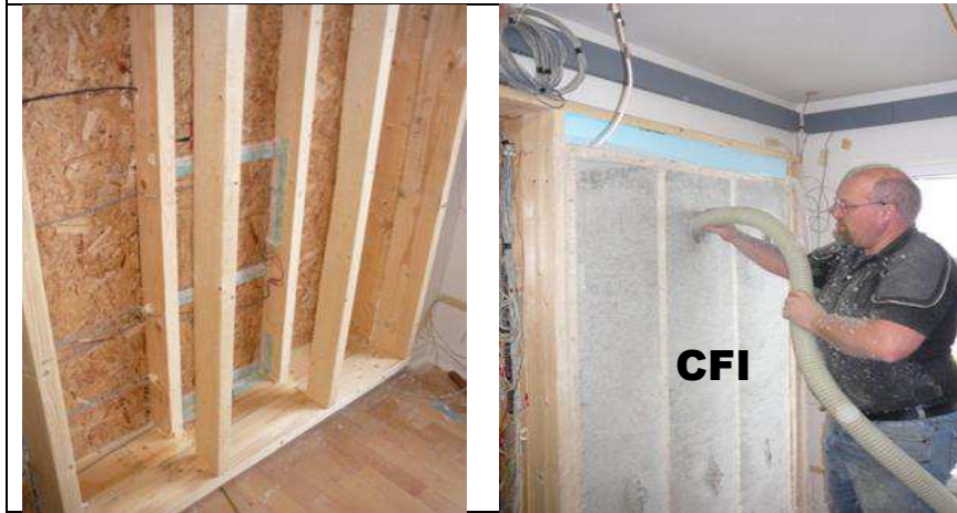
Figure 16. Wall 6 (CFI) Interior wood frame prior to (i) & following installation of cellulose fibre insulation in stud cavities (ii), & PE
