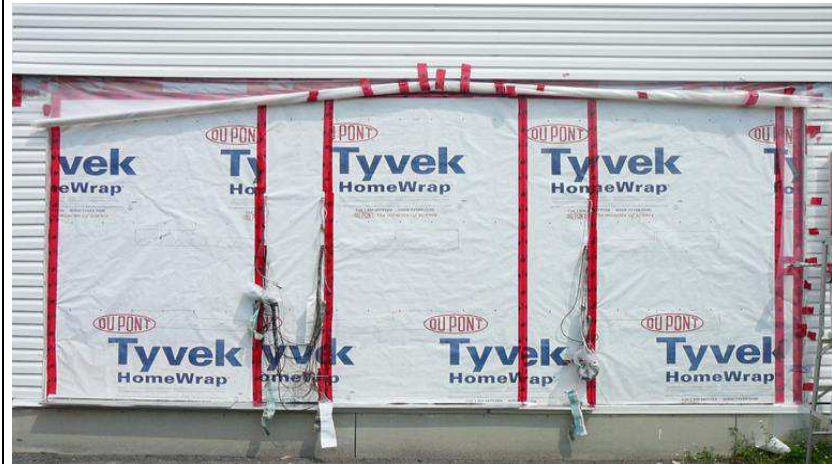
Figure 7. Installation of W1, W2, and W3 in FEWF showing sheathing membrane
