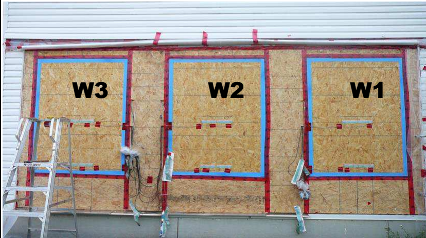
Figure 6. Installation of W1, W2, and W3 in FEWF showing exterior sheathing panel (OSB)
