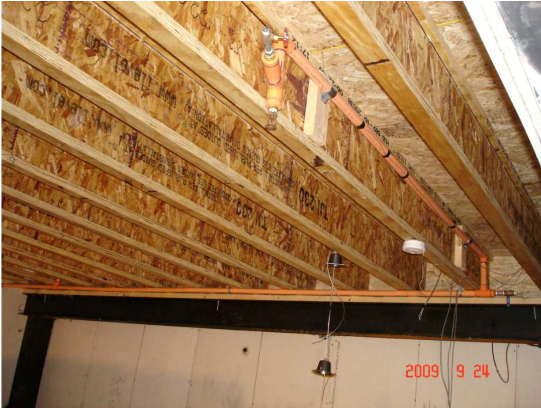
Figure 63. Sprinkler and CPVC piping installation with exposed wood I-joists in Test PF-03
