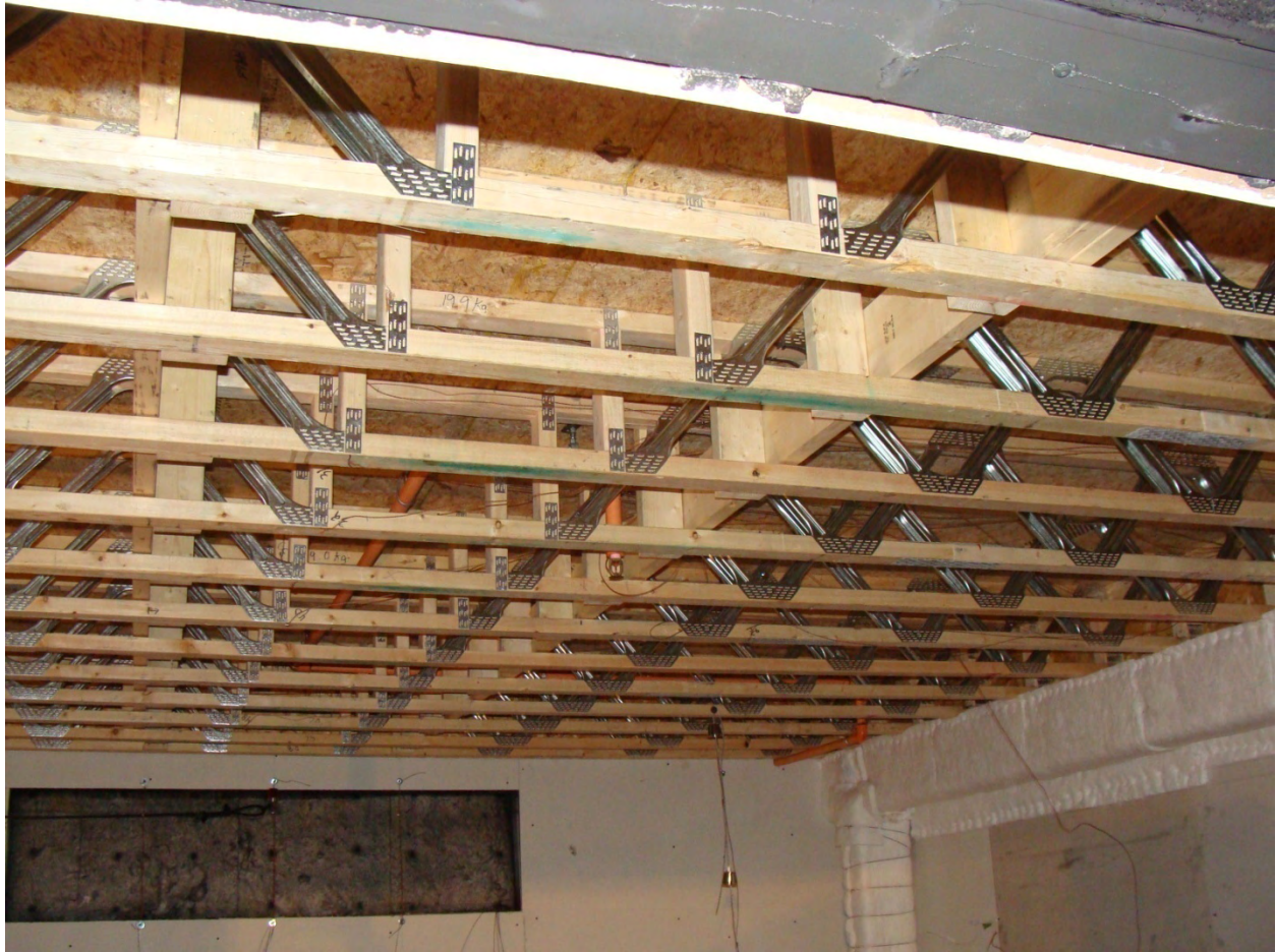
Figure 83. Metal-web wood truss assembly and sprinkler in Test PF-06
