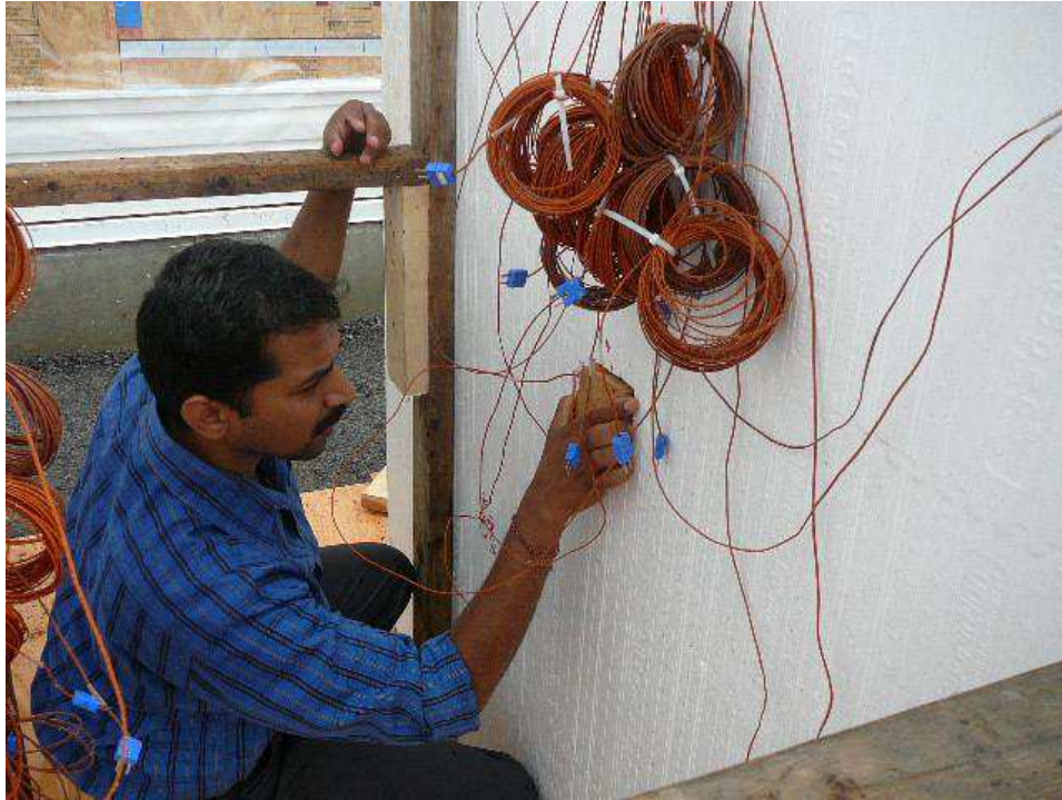
Figure A-56. Replacing the foam block with a piece of wood for the concrete pour.
