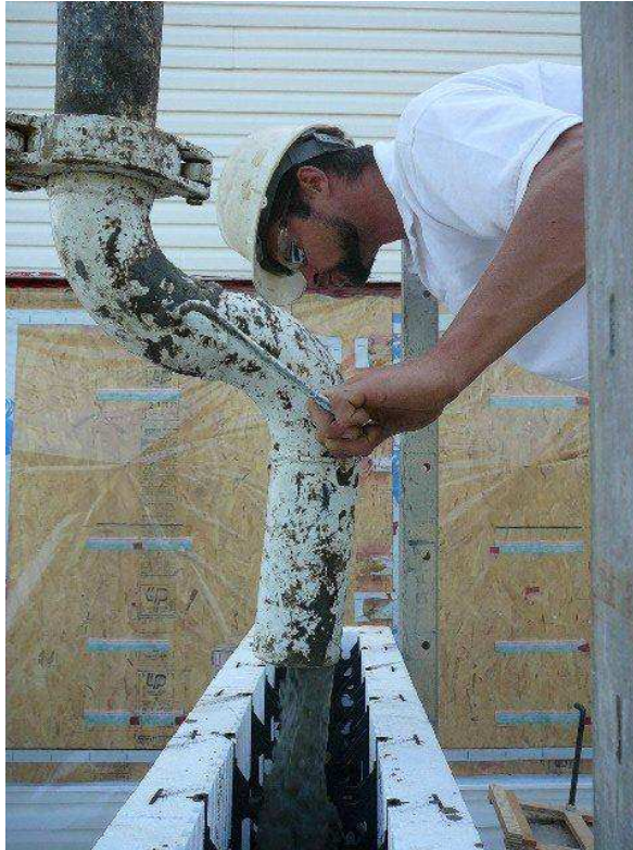
Figure A-11. Pouring the concrete into the insulating form.
