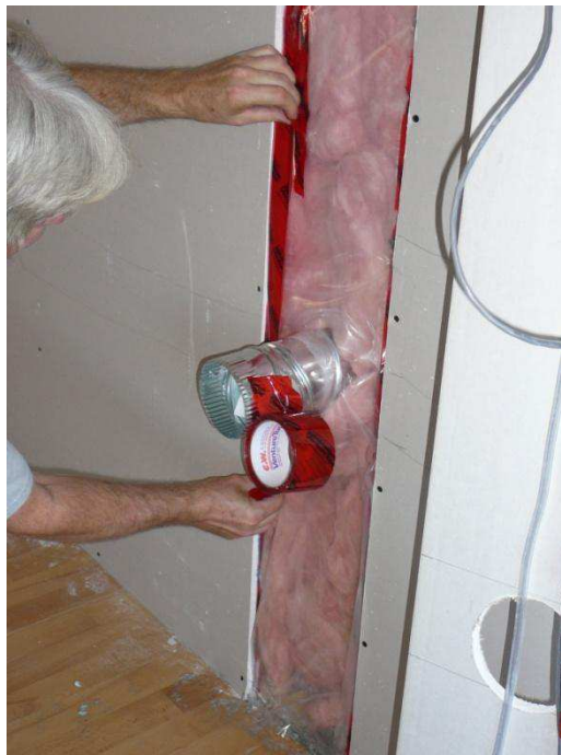
Figure A-46. Tape seals the air/vapour barrier to the surrounding wall assembly. A ventilation duct passes through the wiring chase, to permit air conditioning of the test chamber during the cooling season.
