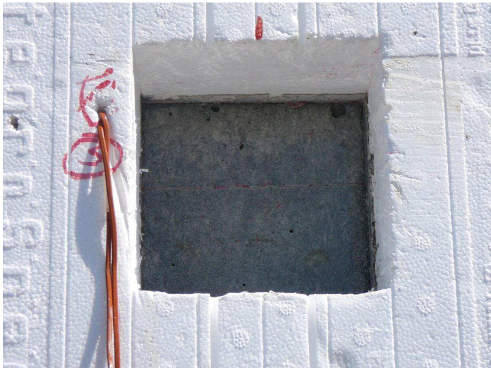
Figure A-61. Cured ICF wall with removed foam block.
