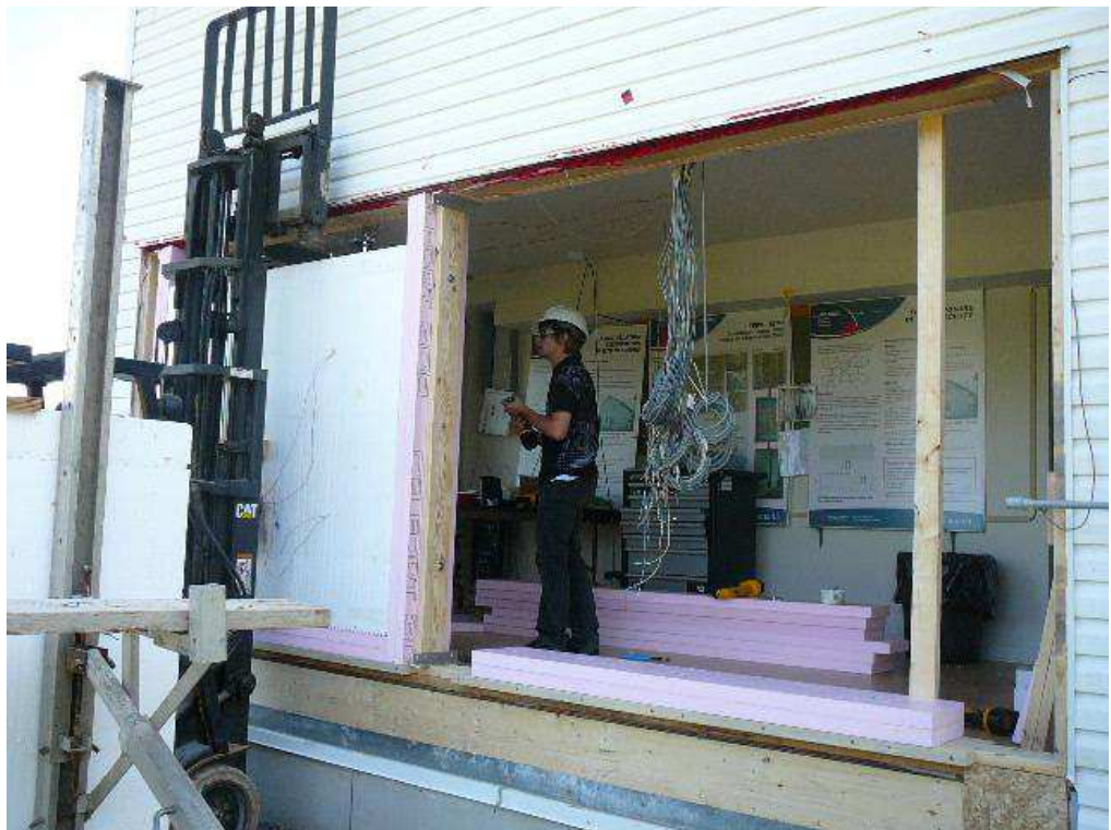
Figure A-21. Lifting the first ICF wall into position.
