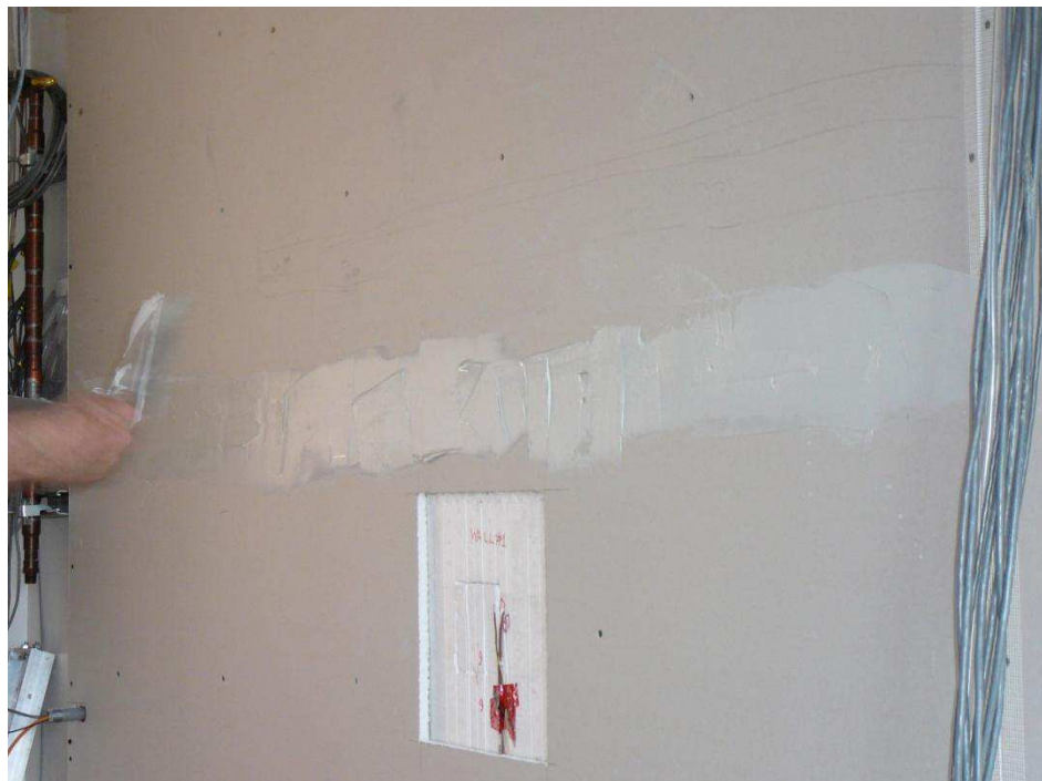
Figure A-47. Installing drywall over the wiring chase between the ICF walls.
