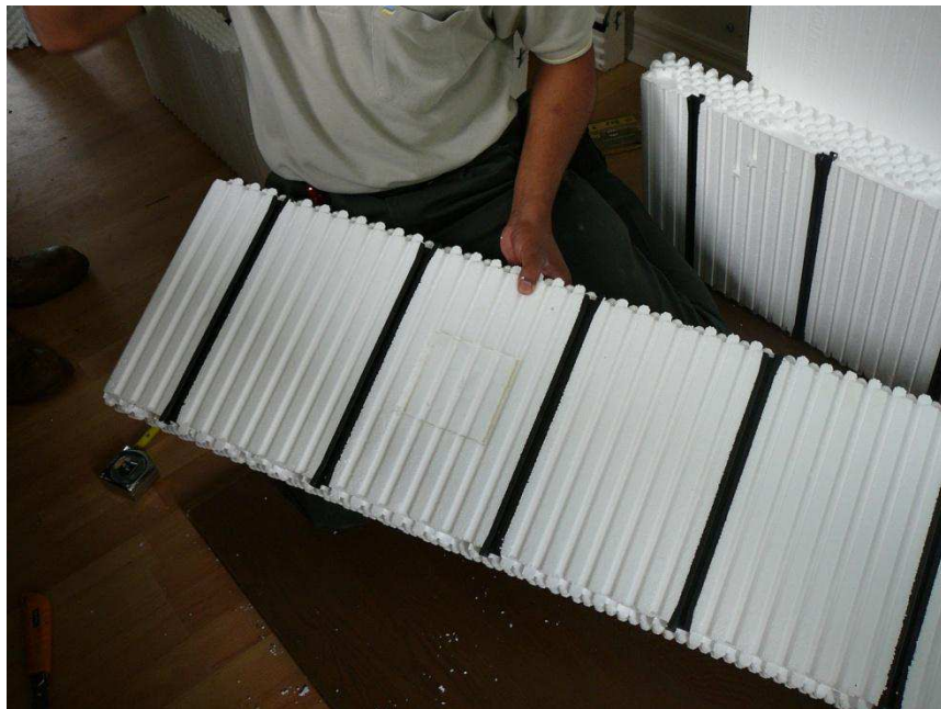
Figure A-55. Removing a block of the EPS foam from the insulating form.
