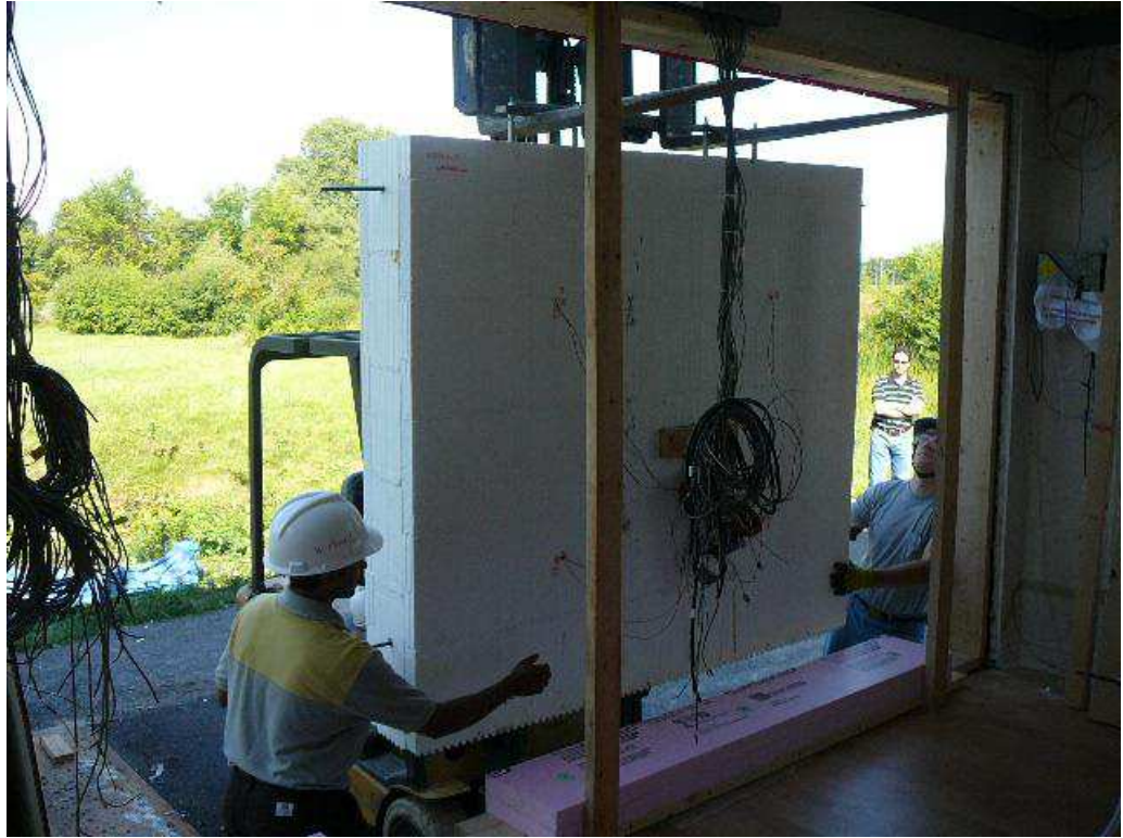
Figure A-20. Lifting the first ICF wall into position.
