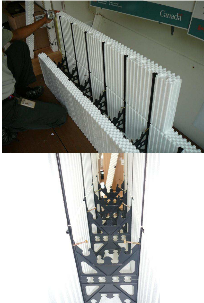
Figure A-3. Assembling the insulating form inside the Research House.
