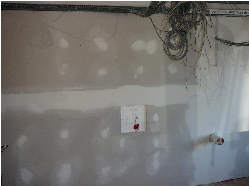
Figure A-49. The seams and screw holes in the wall covered with drywall compound.
