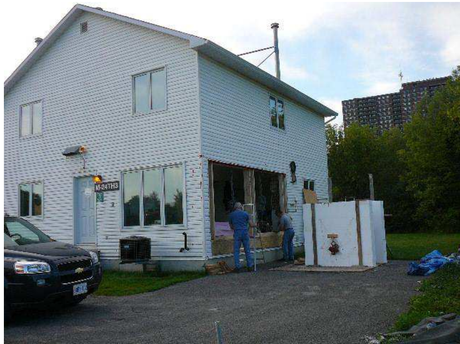
Figure A-18. Preparing the FEWF opening for ICF wall installation.
