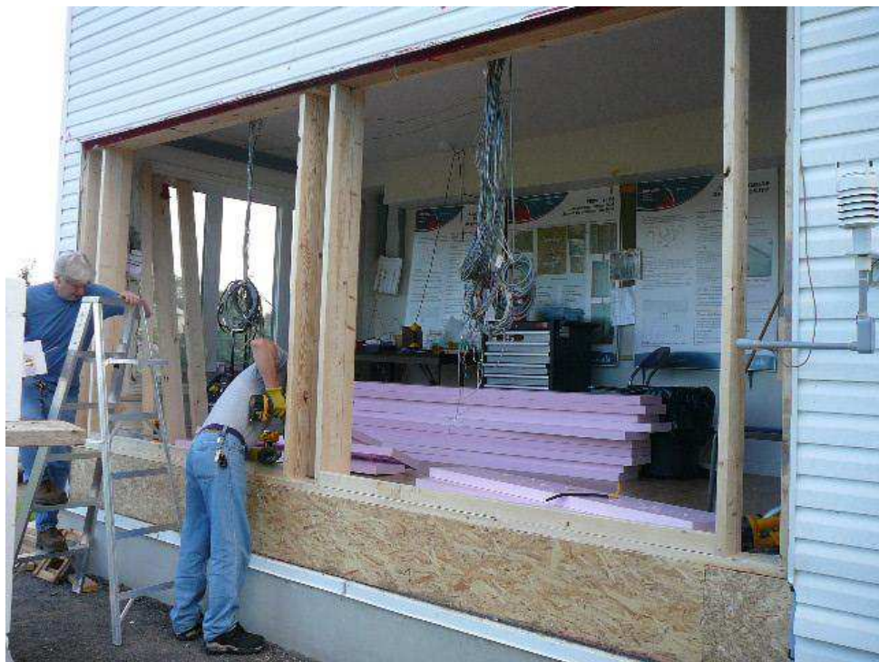
Figure A-19. Preparing the FEWF opening for ICF wall installation.
