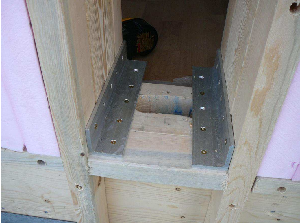
Figure A-30. Metal L brackets hold the framing in place on either side of the ICF.
