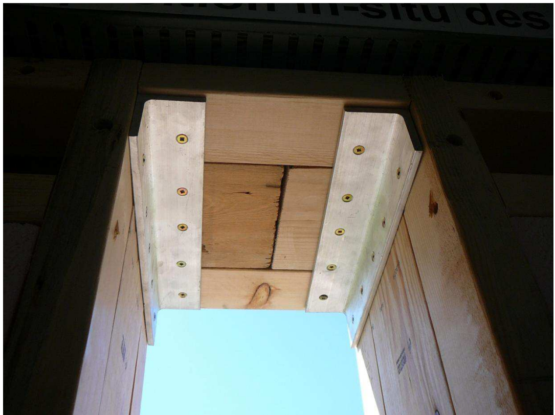
Figure A-31. Metal L brackets hold the framing in place on either side of the ICF.
