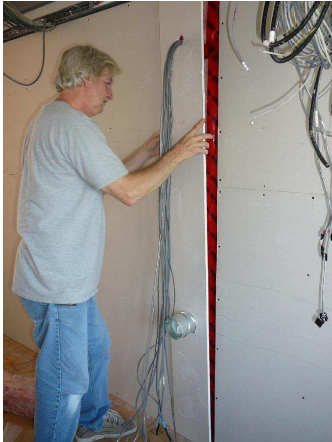
Figure A-47. Installing drywall over the wiring chase between the ICF walls.
