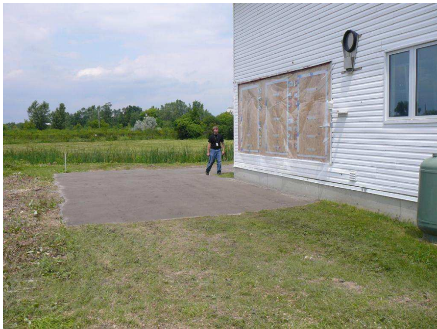
Figure A-2. Installation of a gravel pad to allow the forklift room to manoeuvre when lifting the ICF walls into place.
