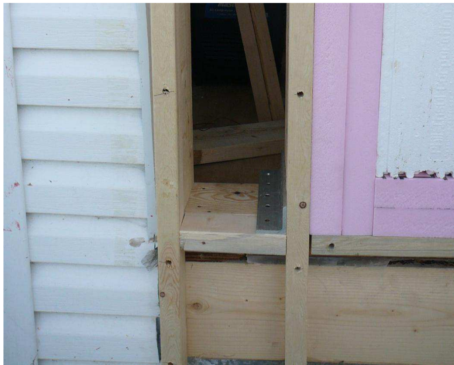
Figure A-29. Metal L brackets hold the framing in place on either side of the ICF.
