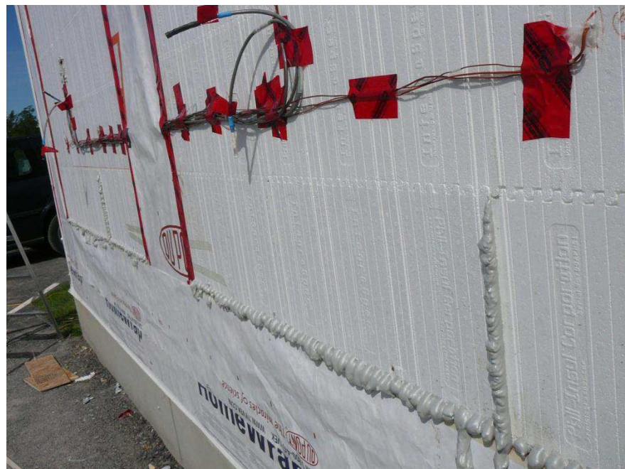
Figure A-36. Gaps in the ICF foam filled with low expansion polyurethane foam. A temporary sheathing membrane skirt prevents foam from adhering to the permanent sheathing membrane.
