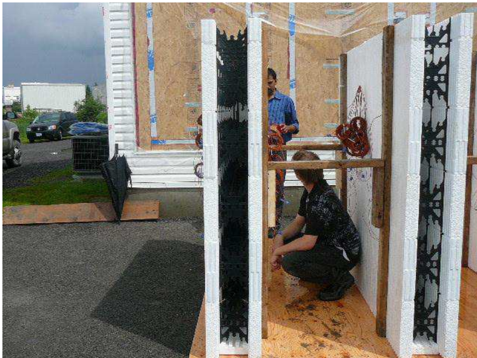
Figure A-6. Preparing the three insulating forms for the concrete pour.
