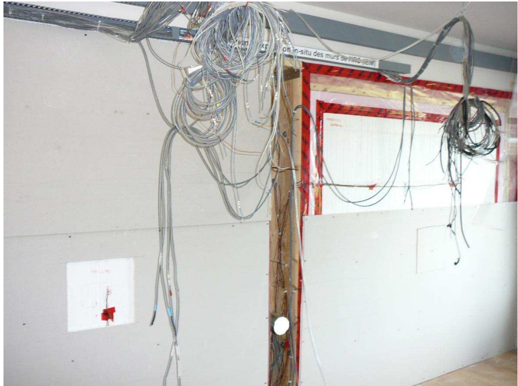
Figure A-43. Drywall being installed on the interior of the ICF wall specimens. A square access panel was cut in the centre of the drywall to allow access to the instrumentation (including heat flux transducers) on the surface of the ICF.
