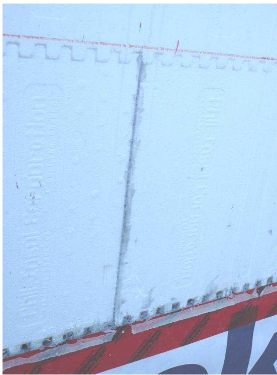
Figure A-38. Excess foam trimmed from the face of the ICF once cured, with the temporary skirt removed.
