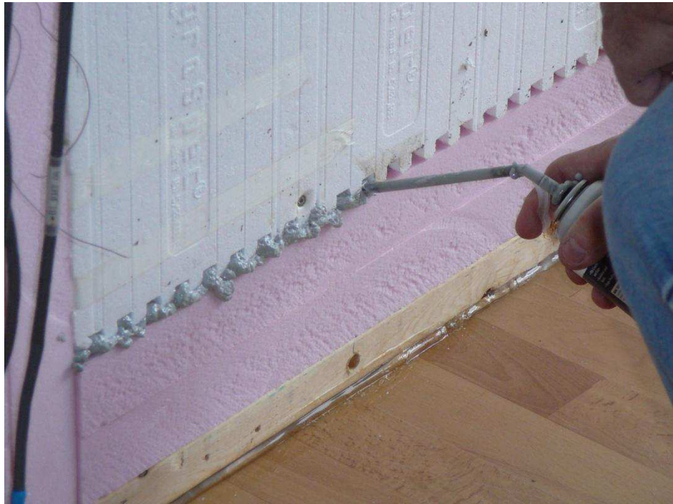
Figure A-41. Gaps in the ICF foam filled with low expansion polyurethane foam. Once cured, excess foam was trimmed from the interior face of the ICF.
