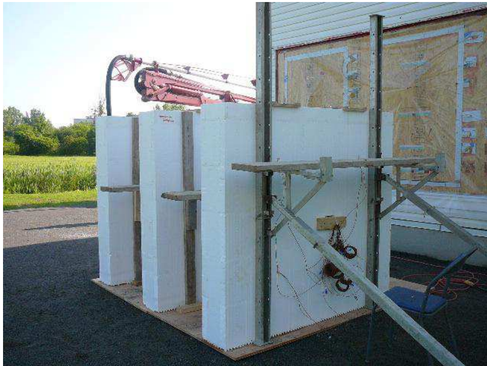
Figure A-9. Preparing the three insulating forms for the concrete pour.
