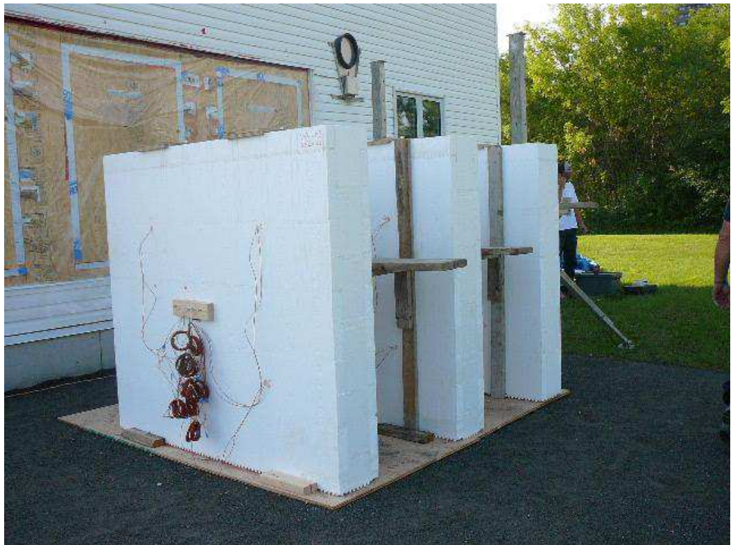
Figure A-8. Preparing the three insulating forms for the concrete pour.
