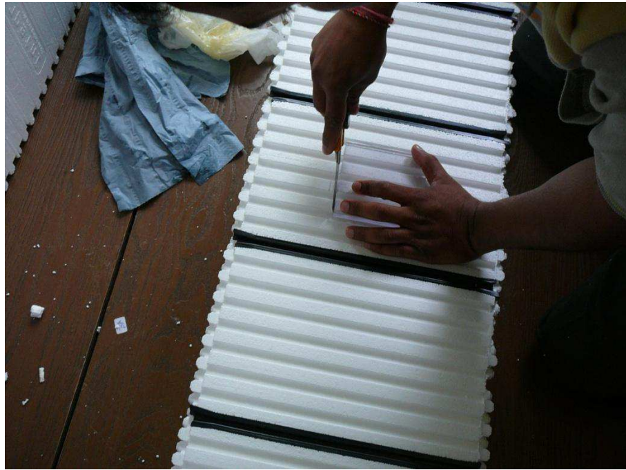
Figure A-54. Removing a block of the EPS foam from the insulating form.
