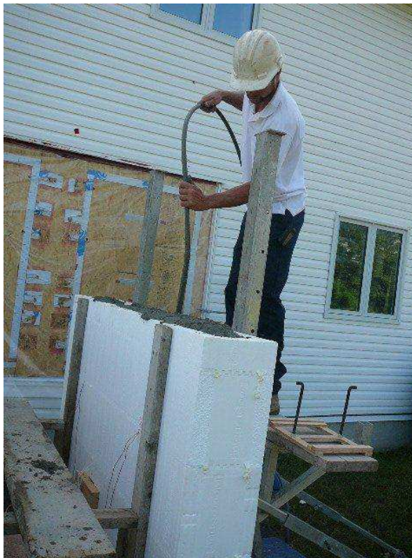
Figure A-12. Vibrating the concrete to remove air pockets.
