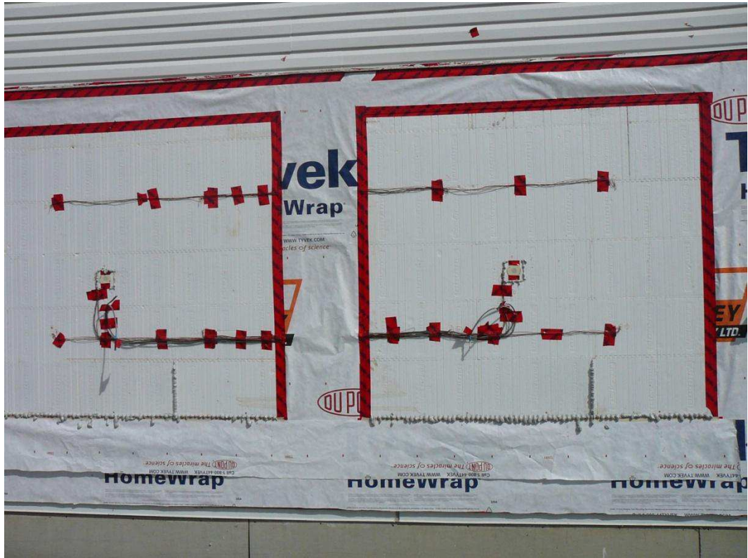
Figure A-37. Gaps in the ICF foam filled with low expansion polyurethane foam. A temporary sheathing membrane skirt prevents foam from adhering to the permanent sheathing membrane.
