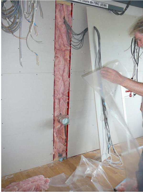
Figure A-45. The wiring chase was filled with glass fibre batt insulation, and sealed with a polyethylene air/vapour barrier.
