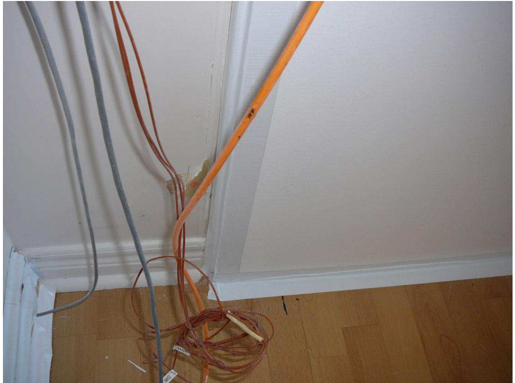
Figure A-51. The edges of the drywall were taped to the surrounding walls, floor and ceiling.
