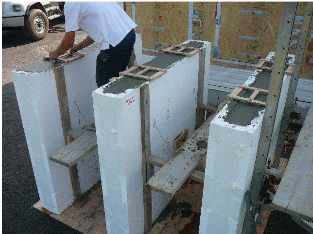
Figure A-16. The alignment jig holds the metal rods in place while the concrete cures.
