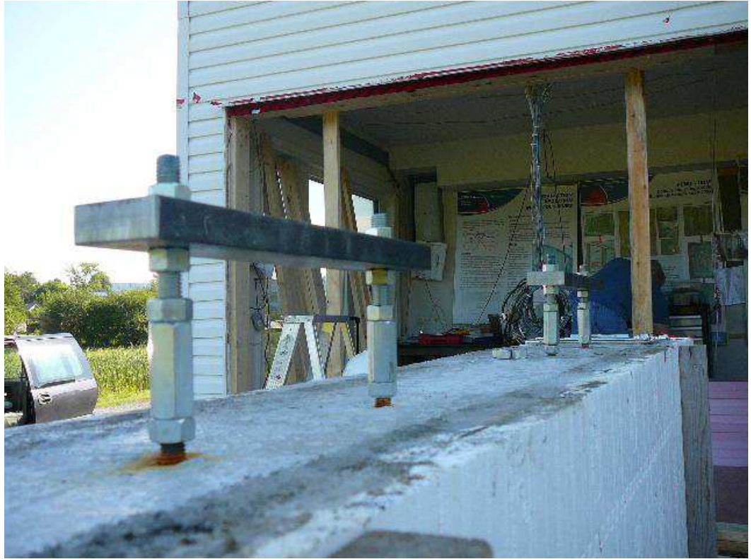
Figure A-17. Once the concrete was cured, the wooded jig was removed, extensions were added to the threaded rods, and metal plates were attached to provide lifting points for the forklift.
