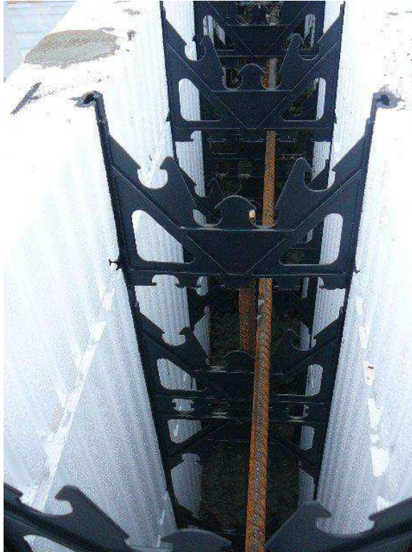
Figure A-7. Steel rebar inserted into the ICF frame prior to pouring the concrete.
