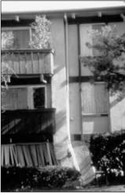
**Figure 2.** Excessive deformation of a weak first storey in an apartment building, Northridge earthquake 1994. In another part of the building the ground floor collapsed completely.
