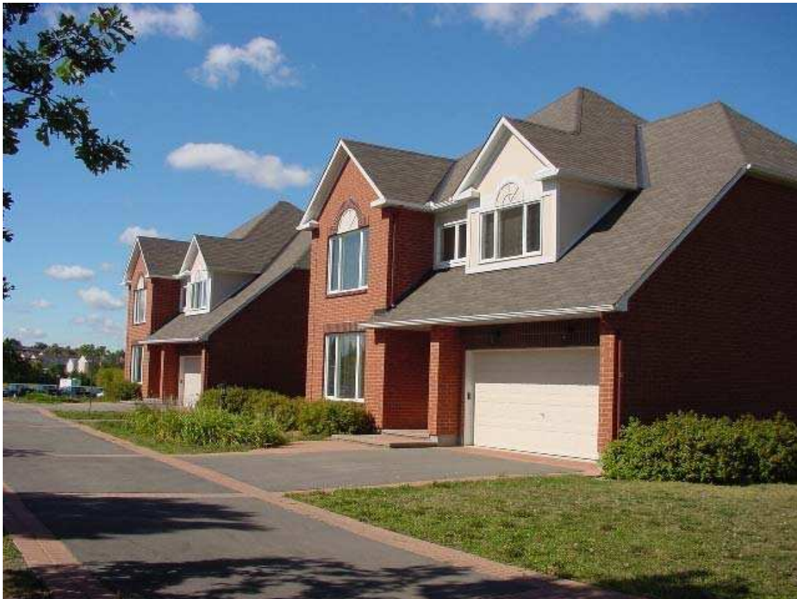
Figure 1 - CCHT Twin Research House Facility
