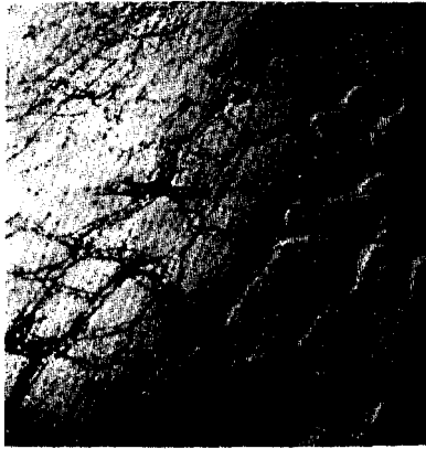
Fig. 10. Frost damage on a heavy old surface in the form of a random pavement mosaic occurring under heavy truck traffic. Broad crack zones in a pavement which has become brittle.
