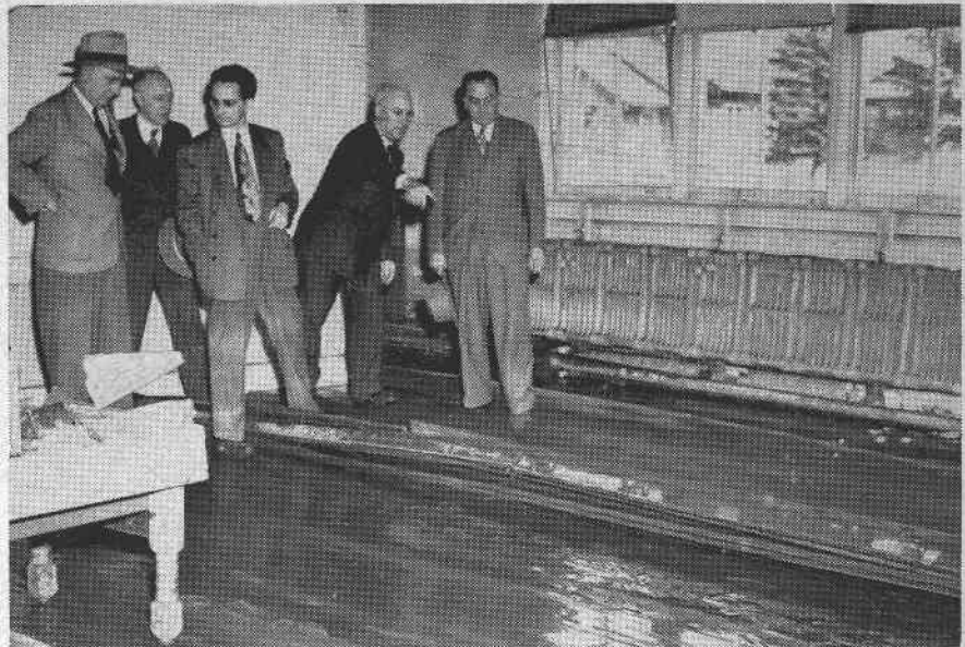
WINNIPEG School Board members inspect flood damage to a Winnipeg school.
