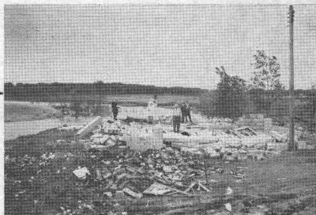
Complete destruction of walls of hollow concrete blocks.
