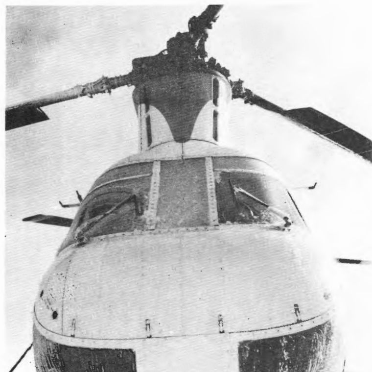
RUN 202-2 WINDSHIELD ANTI-ICING IN FREEZING RAIN
