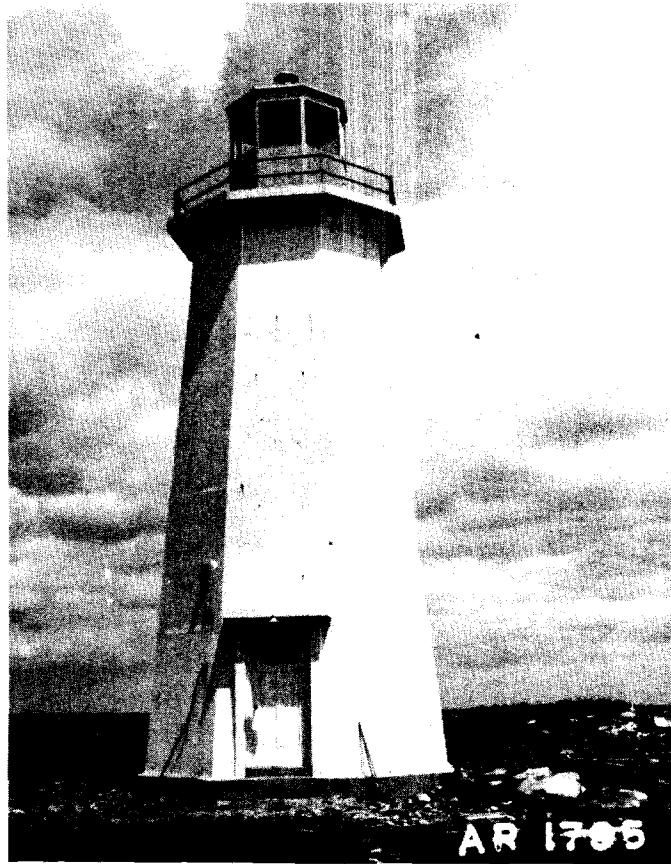
FIGURE 24a Mildew - Southeast Exposure (Cape Roseway - Building 1)
