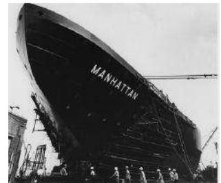
Fig. 13. The icebreaking bow of the *Manhattan* being installed prior to her voyages through the N-W Passage in 1969 and 1970.
