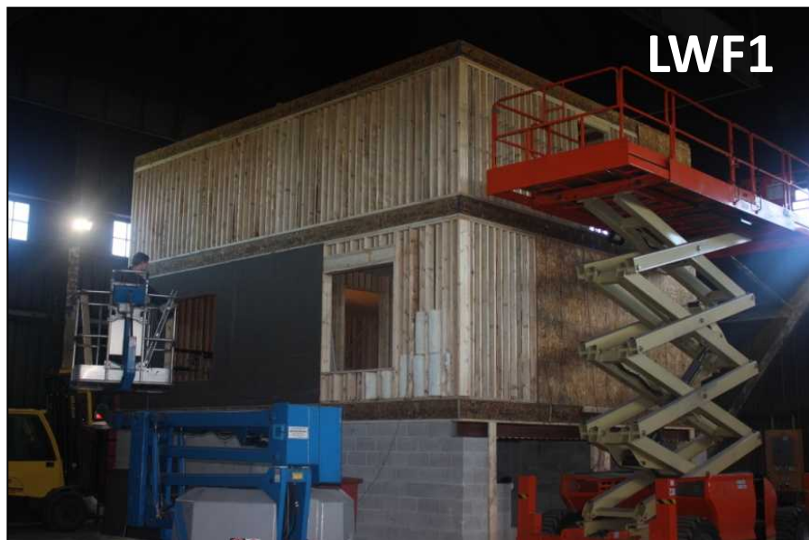
Figure 29. Large-scale apartment test structures under construction.
