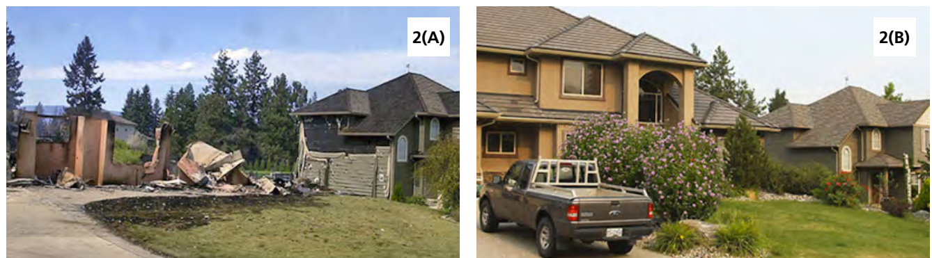
Figure 2. (A) Street-level photo from immediately after the fire shows that buildings immediately adjacent to destroyed houses are not wholly untouched. Note the melted vinyl siding on the green house. (B) The same two lots, showing the nearby house repaired and the destroyed one rebuilt. It appears the new house has been rebuilt with non-combustible stucco exterior finish. (A and B: Ottawa Citizen 2013).
