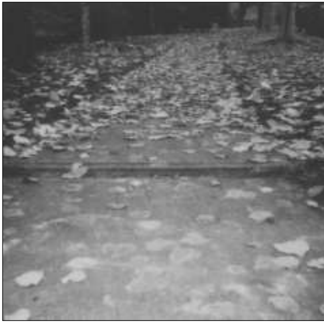
Figures 5a and 5b. Sidewalk before and after mud jacking repair of a fault.
