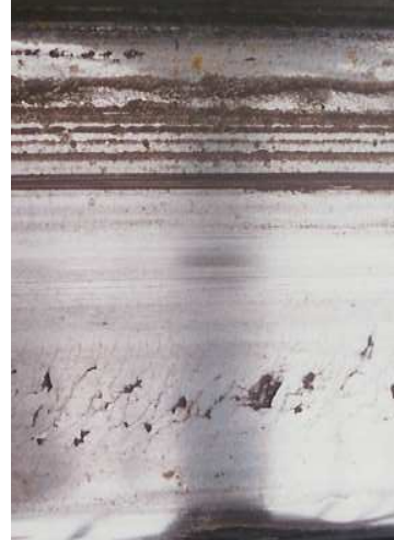
F) Deeper cracks on the field/rim side of the wheel tread with material starting to shell.
