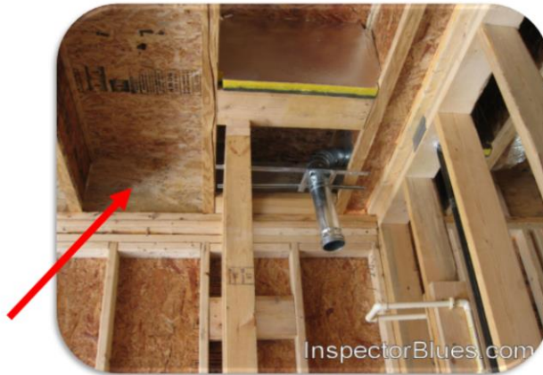
Fire block at wall
