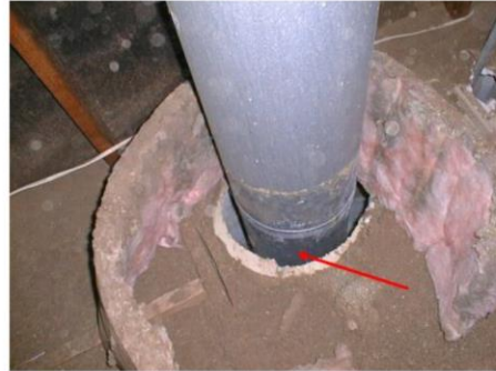
Semi-rigid mineral fibre fire stop
