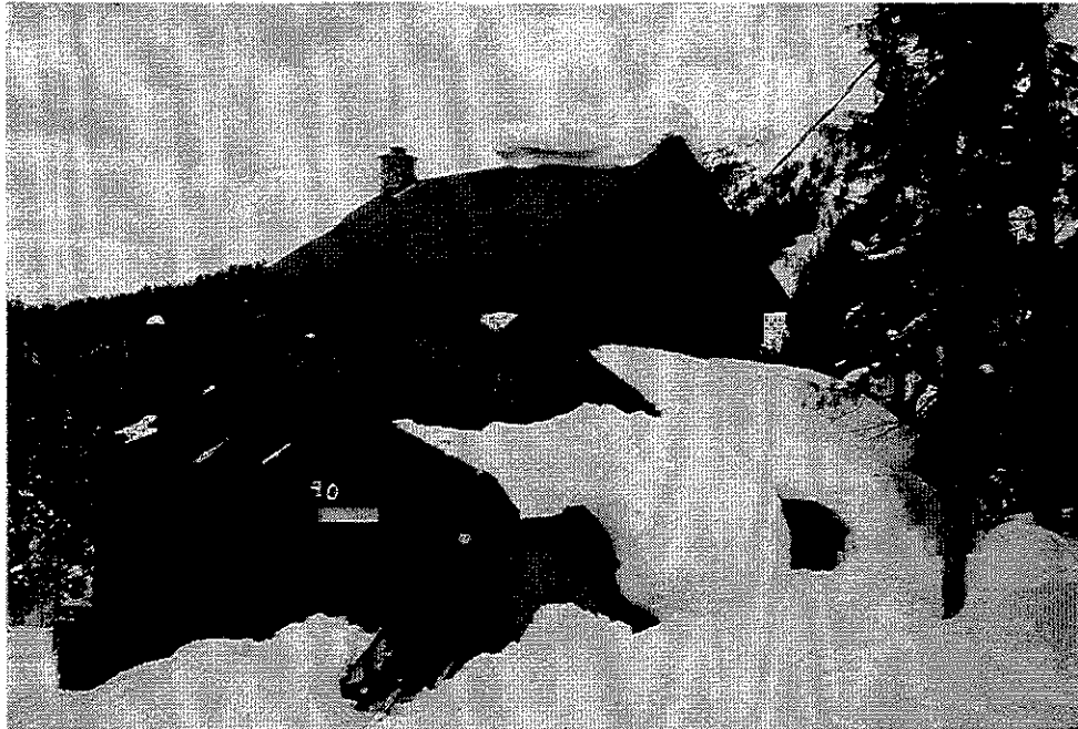
Figure 16. Slippery metal roof has shed snow. Notice "hat" of heavy snow at ridge posing danger below.
