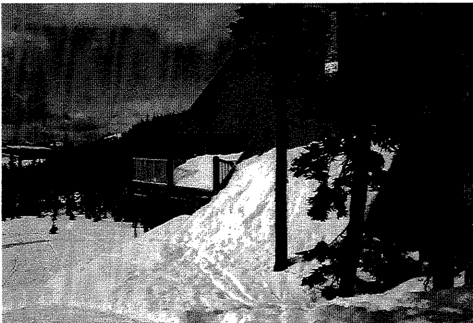
Figure 19. Railing around deck broken or removed to prevent breakage by sliding snow.
