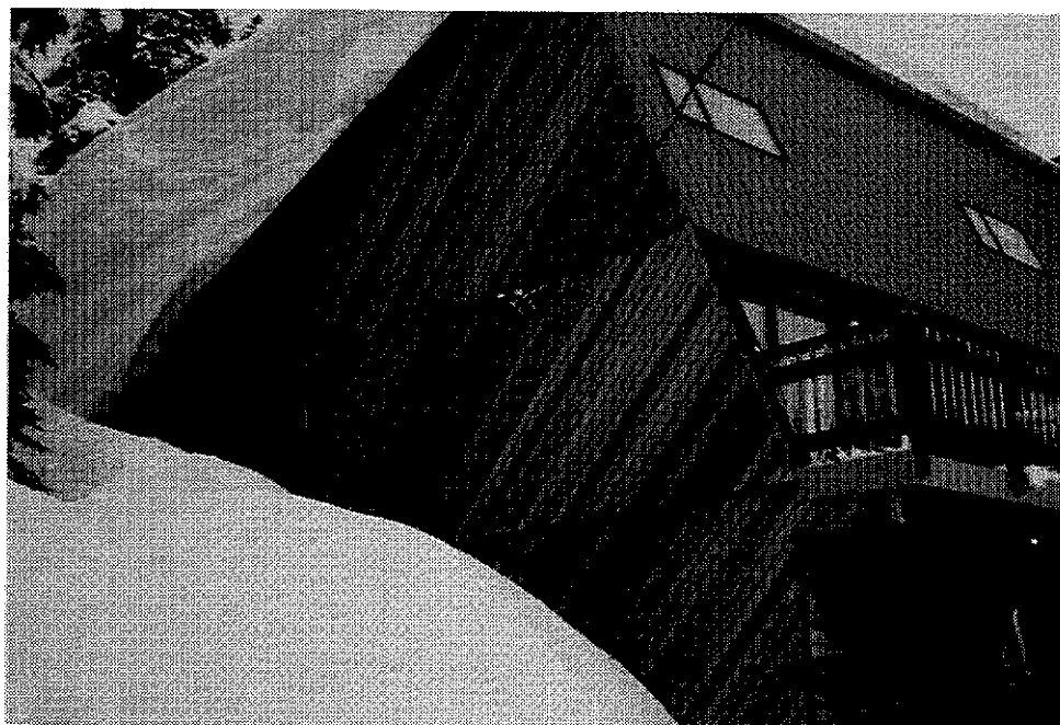
Figure 5. Condominium 81, April, 1983. Very deep snow cannot slide off because the roof slopes towards the hill.
