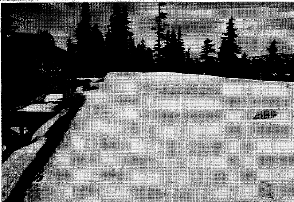
Figure 15. Perimeter of flat roof cleared by snow blower kept on roof.
