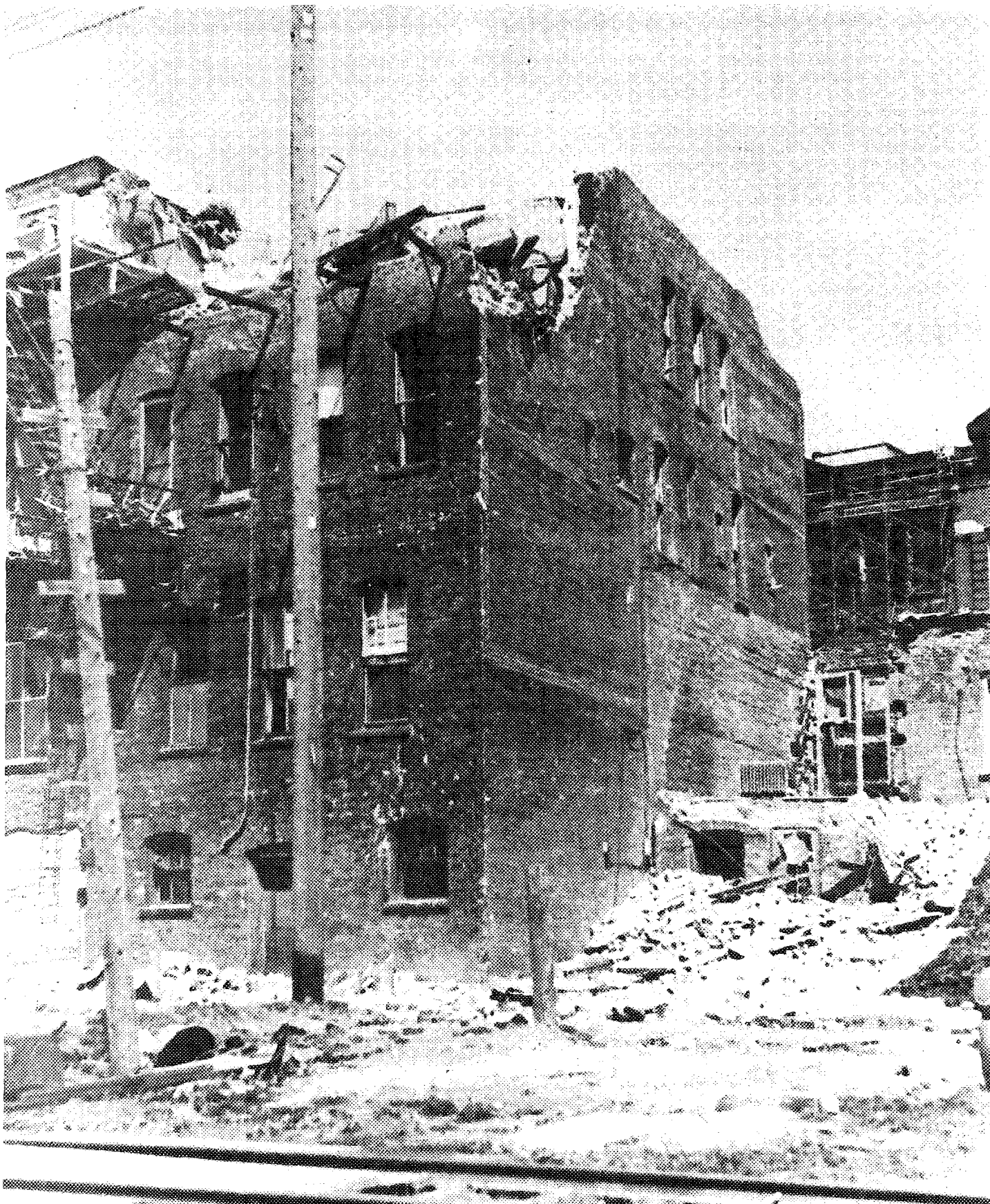
Figure 4 Damage to old building of masonry bearing wall type along waterfront (note bicycle still on third floor)
