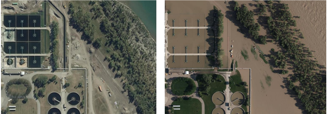
Figure 4-7 Flooded wastewater treatment plant in Calgary, AB (Source: City of Calgary https://maps.calgary.ca/riverflooding/ )
