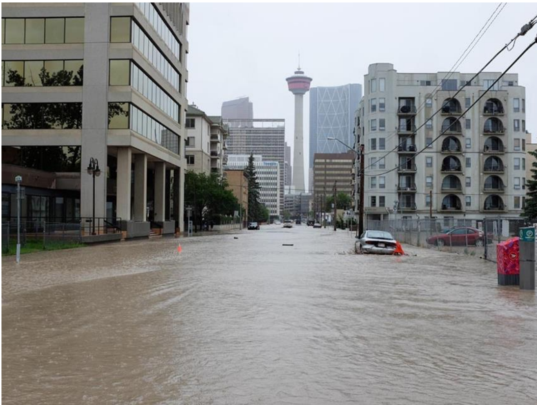
Figure 4-2: Energy and financial buildings surrounded by flood water in Calgary, Alberta (source: Jen Gerson/National Post).
