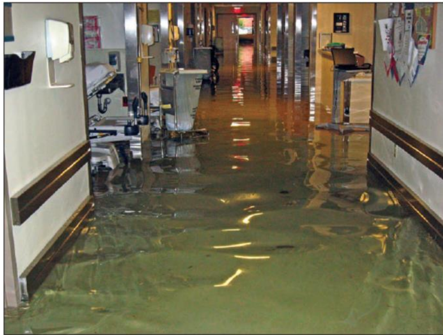
Figure 4-6: Flooding in New Jersey Hospital – Hurricane Sandy (source: FEMA)
