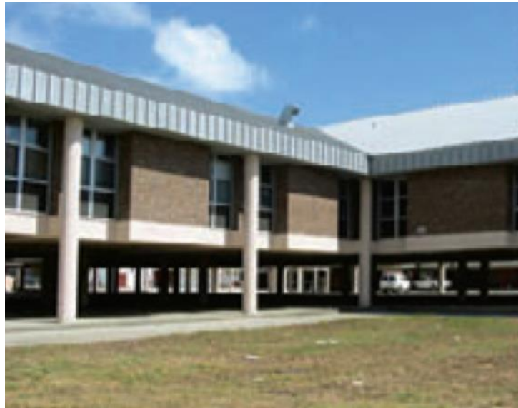
Figure 4-4: Elevated school building (source: FEMA 424)
