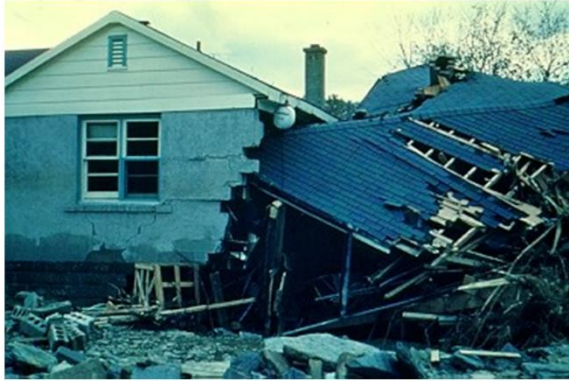
a) House floated into house (source: https://www.canada.ca/en/environment-climate-change/services/water-overview/quantity/floods/events-ontario.html )
