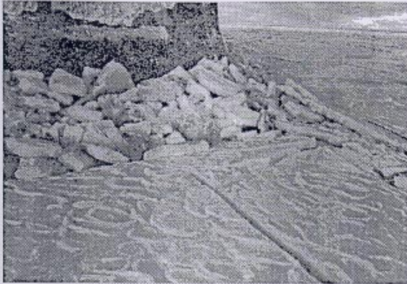
Figure 5.16: Prior to the formation of grounded ice rubble around the caisson and prior to the onset of landfast ice conditions, the moving ice cover failed against the Molikpaq's sloped sides in bending, at low load levels.
