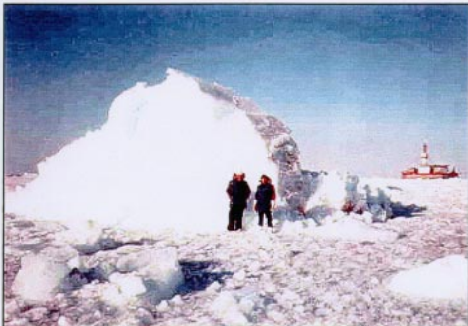
Figure 5.7: The upper photo shows multi-year ice crushing against the Molikpaq on April 12th where the ice extrusions caused by ice clearance can be seen, while the lower photo shows representative ice extrusion debris that has been turned back by the ice deflector.
