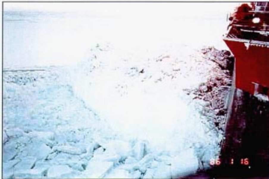
Figure 3.11: Typical examples of ice rubble that formed off the Molikpaq caisson. The upper photo shows a floating rubble formation while the lower photo shows a grounded rubble pile. When the Molikpaq's deployment draft was deep, the occurrence of grounded rubble piles was very rare and they would be swept away by subsequent ice movements anywhere from a few hours to a few days after they had formed.
