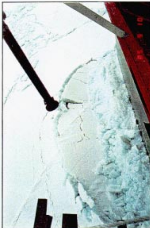
Figure 3.7: Typical examples of flexural ice failures. The upper figure shows bending failures at the ice sheet's leading edge, while the lower figure shows downwards bending due to the weight of the rubble debris at the caisson wall.
