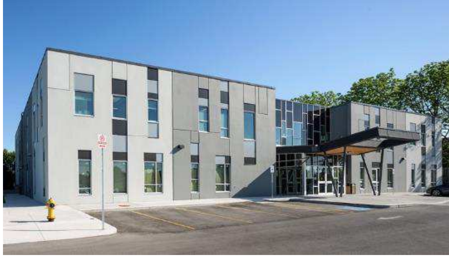
Figure B.19: Example of a PCW building ( http://www.tilt-up.org/projects/profile/?id=5484 )
