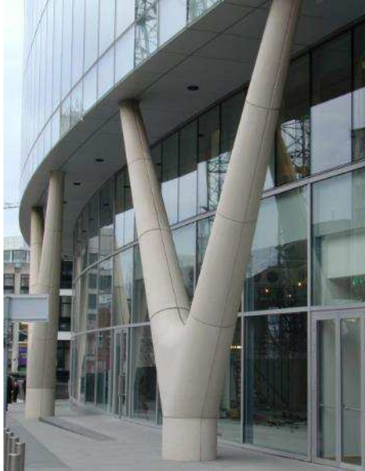
Figure B.22: Typical precast concrete cover on a steel or concrete moment frame ( https://www.buildingdesignindex.co.uk/entry/110238/BCM-GRC/GClad-glassfibrereinforced-concrete-column-casing/ )
