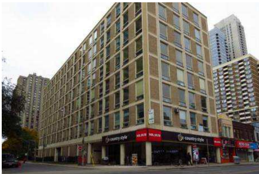
Figure B.17: An example of a CIW building showing concrete frame and infill masonry shear walls ( https://thetorontoblog.com/ )
