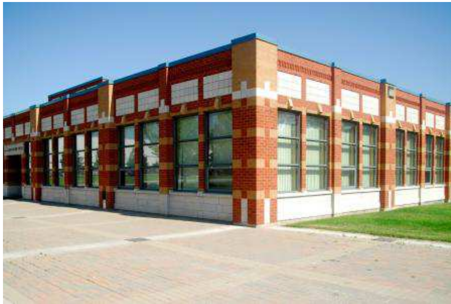
Figure B.27: An example of a reinforced masonry bearing wall building ( http://www.canadamasonrydesigncentre.com/about/our-staff/ )
