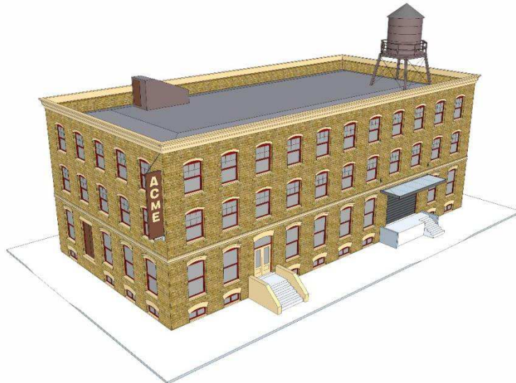
Figure A.11: A building with parapets and other falling hazards including a canopy over a loading deck and a water tank on the roof (from FEMA P-154 2015)
