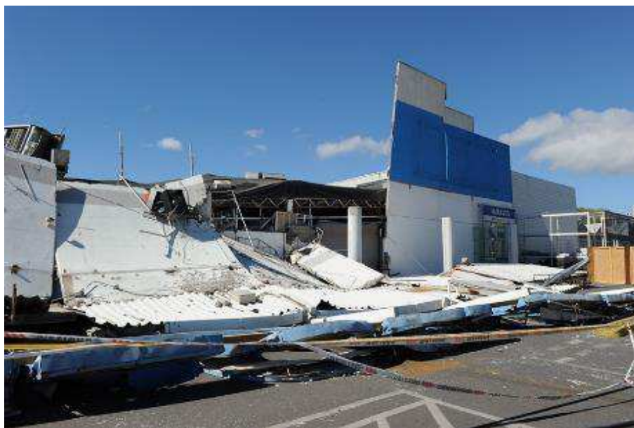
Figure B.20: Collapse of a PCW building ( http://www.reidmiddleton.com/reidourblog/earthquake-reconnaissance-trip-chile/ )
