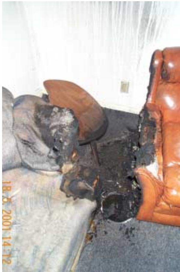
Figure 26. Pictures of the living room after Test 4.
