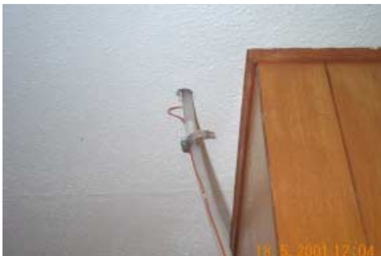
Figure 24. Furniture, ignition source and exposed pipe in the living room.
