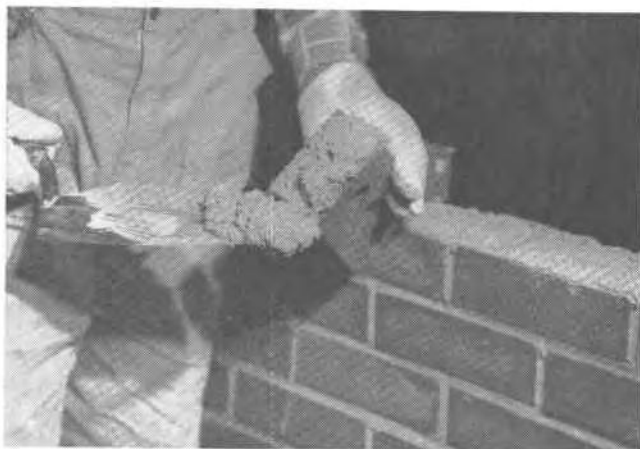
FIGURES 1 AND 2: Place sufficient mortar on end of brick to fill joint completely.
