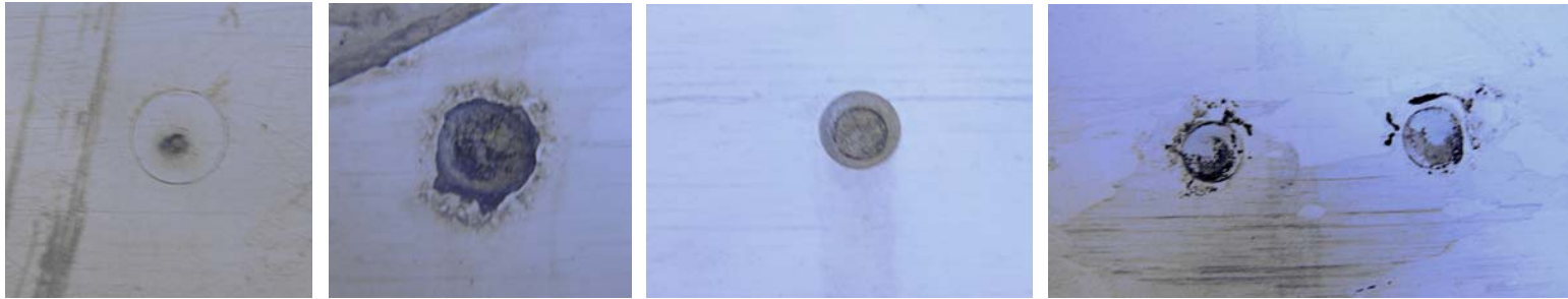
M15 (failed 02/12/2004) M 44
