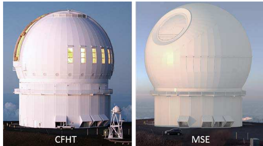
Figure 1: Exterior views of CFHT (ventilation modules open) and MSE (ventilation modules closed).
