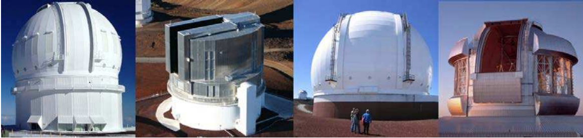
Figure 14: Enclosure styles. From left to right: CFHT, Subaru, Keck, Gemini.
