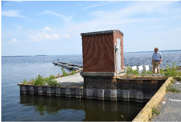
Figure 12: The Pointe-Claire station in August 2022. [Photo: P. Barrette, NRC]
