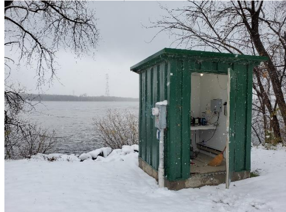
Figure 13: The Lasalle station in November 2022. [Photo: J. Lefebvre, ECCC]
