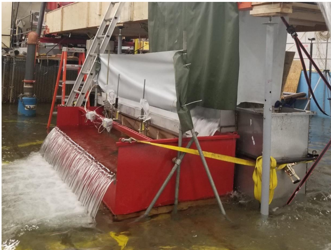
Figure 7. Settlement and Measurement Tanks
