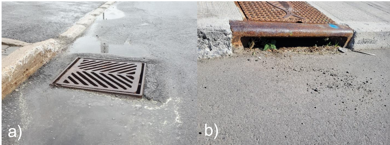
Figure 18. Catch basin a) cover and b) curb mounted inlet installed in a roadway
