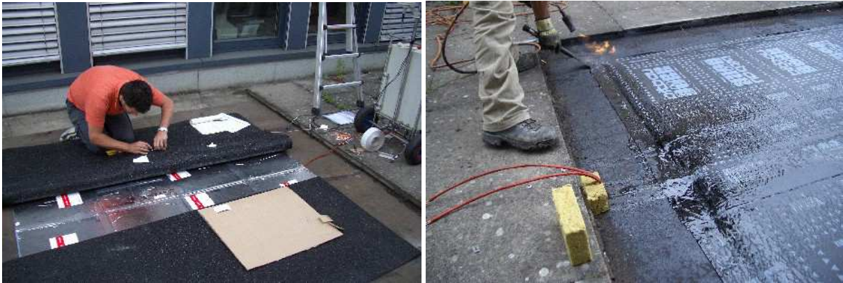
Figure 94: Installation and equipment of a VIP area on a flat roof.
