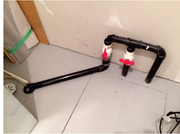
Figure 3e: Freeze Protection for Sump Pump System (Edmonton, Alberta)
