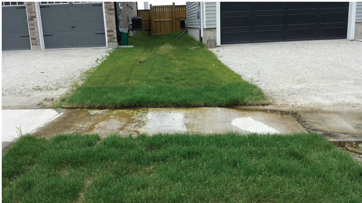
Figure 3b: Saturated Yard Resulting from Sump Pump Discharge (Collingwood, Ontario) 39
