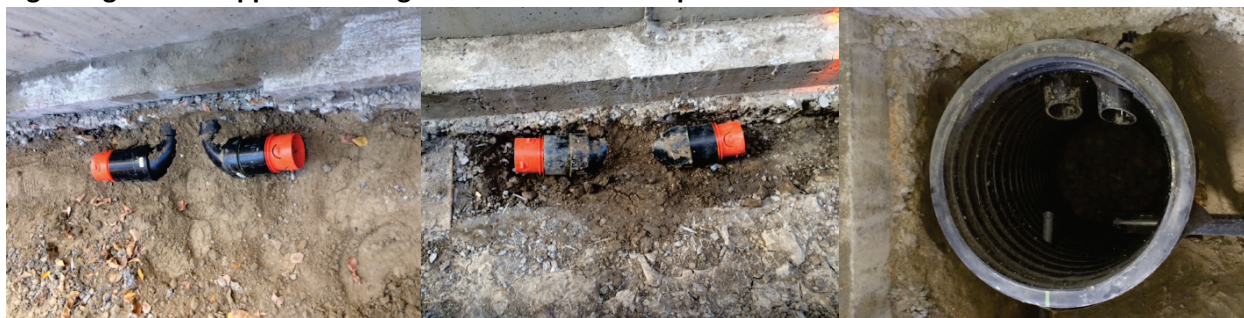
Figure 2g: Access Approach Using Two Outlets in a Sump Pit CC
