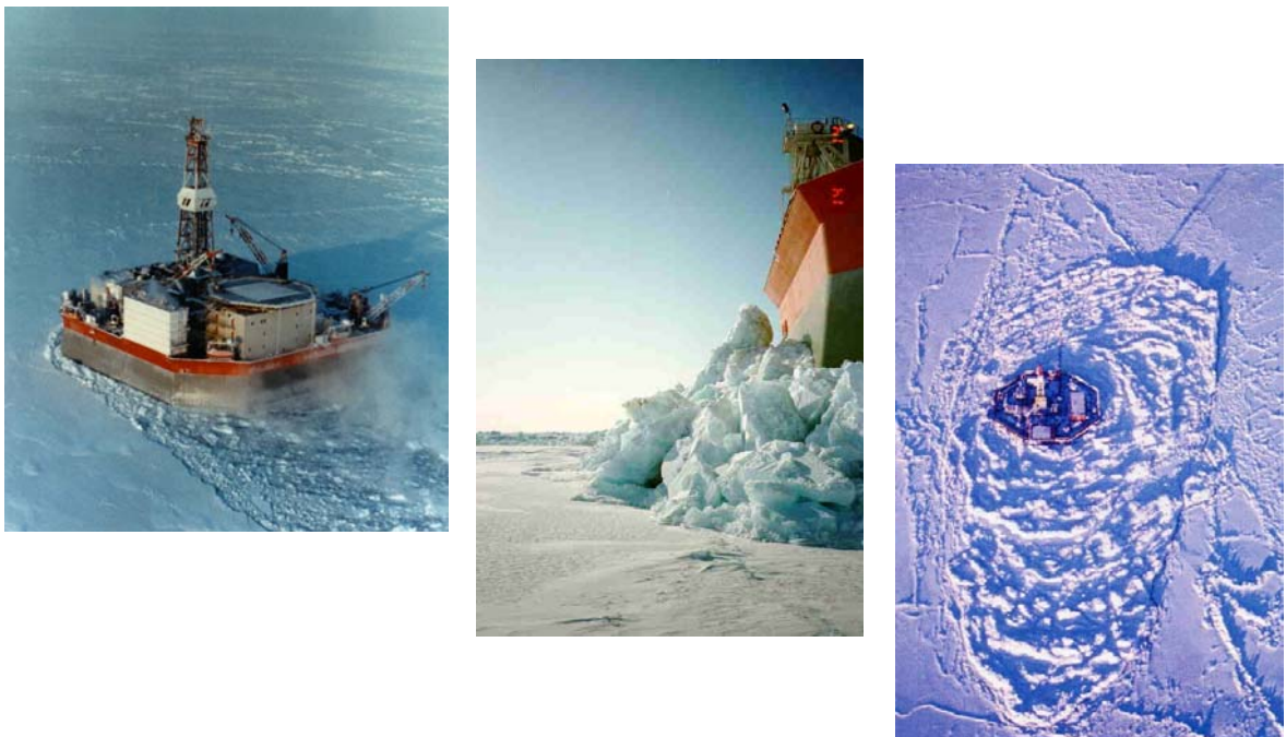
Figure 4.12: Views of the Molikpaq in moving winter pack ice in the Beaufort Sea's transition zone. Because no grounded ice rubble fields formed around this caisson when it was deployed at deep draft (20m), it experienced direct ice action against it, including a few multi-year ice interaction events.
