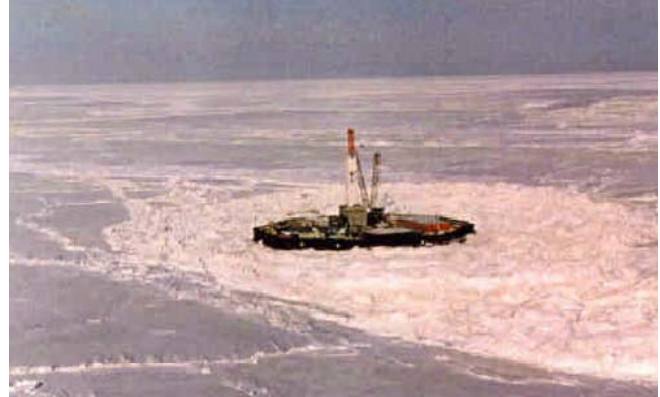
Figure 4.12: Views of the Esso CRI and the grounded ice rubble fields that formed around it.
