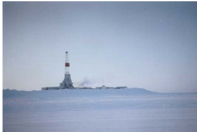
Figure 4.15: Views of the spray ice pads used as drilling platforms in the Beaufort Sea.
