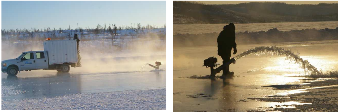
Figure 4: Left) A vehicle fitted with an auger at the back. Right) A pump in action.
