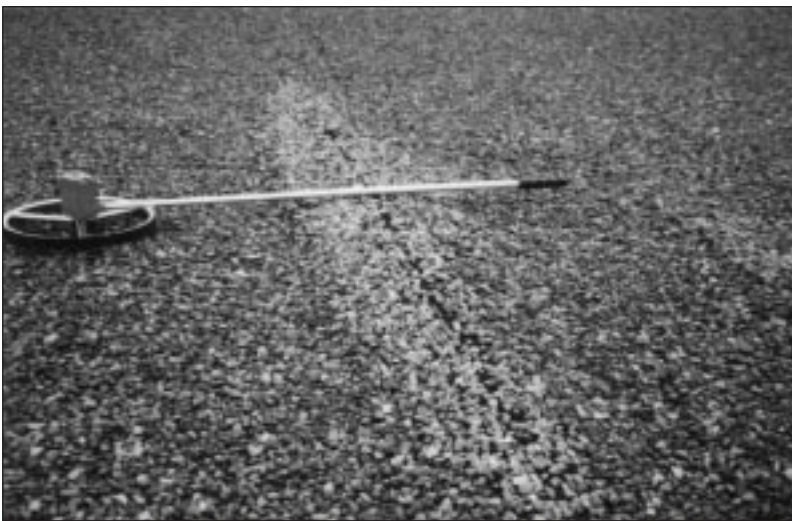
Figure 1. Blistering occurs when pockets of air and moisture trapped between the plies of the membrane, or between the membrane and substrate, expand and displace the membrane.
