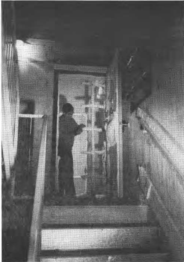
Figure 3 Velocity pressure tubes at open stair door
