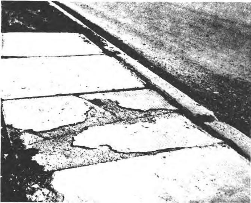
FIG. 1.— Photograph of concrete slab.
