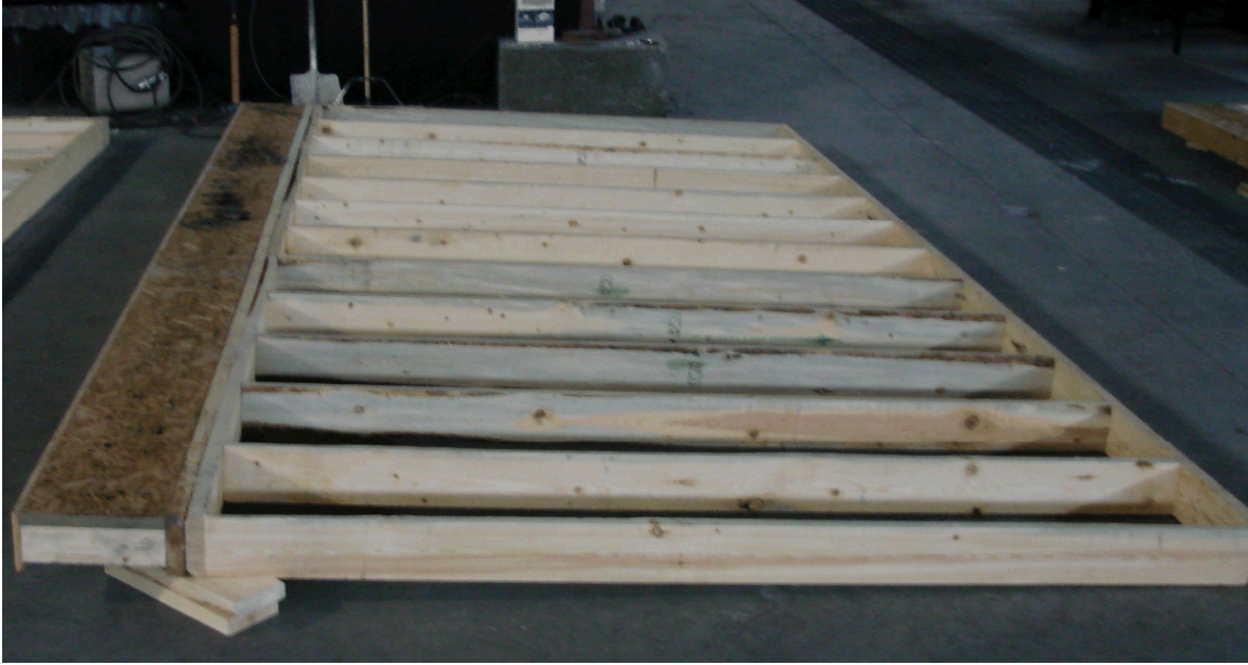
Figure 4. Segment of Wall System under Construction.
