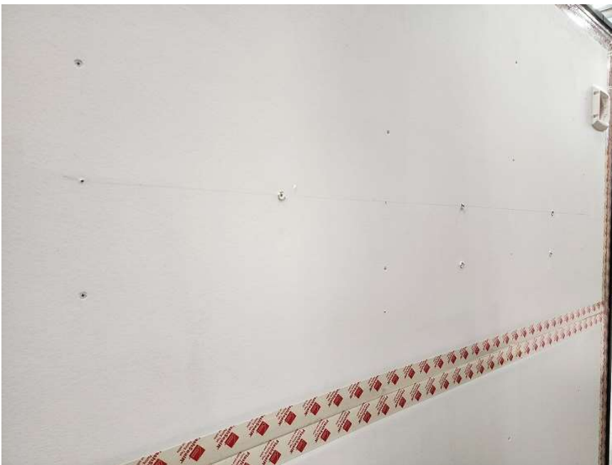
Figure 21. Specimen 7 construction photos
