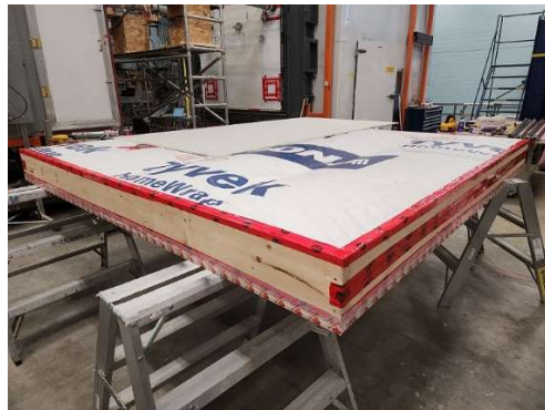
Figure 16. Specimen 2 construction photos
