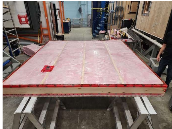
Figure 20. Specimen 6 construction photos
