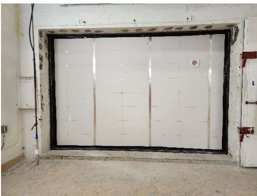
Figure 46. Specimen A1 and A2 construction photos
