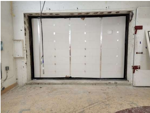
Figure 47. Specimen A3 and A4 construction photos
