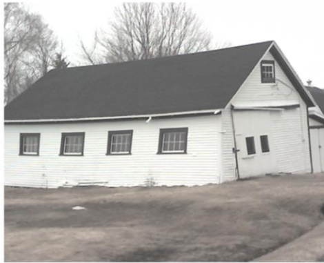
Racking failure
