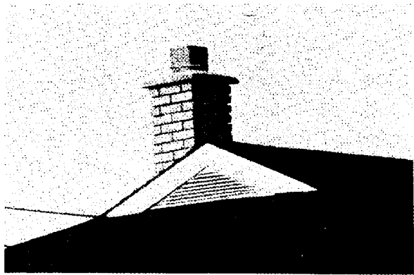
Figure 11. Triangular vent near the ridge of a hip roof
