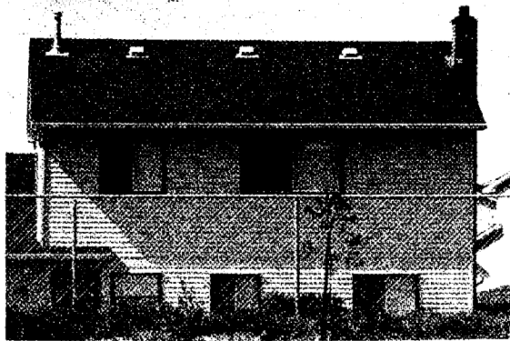
Figure 10. Roof vents near the ridge of a gable roof
