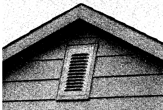
Figure 13. Rectangular vent in a gable roof
