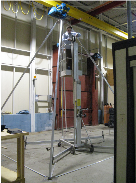
Figure 17: Installing the encoders
