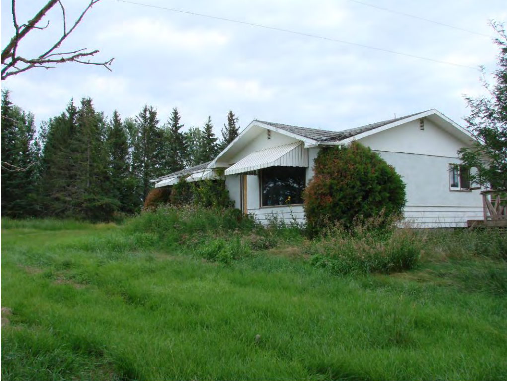
Figure 1. View from driveway showing West side of house.
