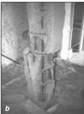
Figure 1. View of (a) normal-strength concrete column and (b) high-strength concrete column after fire-resistance tests
