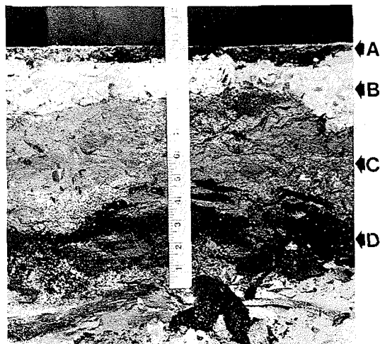
FIG. 1. Section through floor into underlying shale (scale in inches, 1 in. = 2.5 cm). (A) Tiles and bitumen; (B) toplayer of concrete; (C) mushy concrete; (D) weathered shale.
