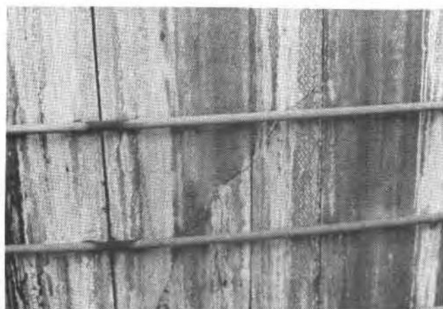
Figure 7c. Effects of structural distortion on silo: Diagonal cracks in staves.
