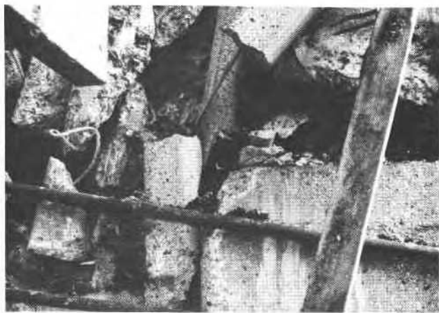
Figure 15. Port Elgin silo, condition of staves in collapsed silo, showing deterioration from acid attack. Photo courtesy H.E. Bellman, OMAF, Walkerton, Ont.
