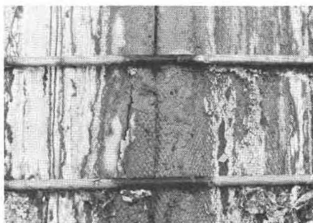
Figure 7d. Effects of structural distortion on silo: Vertical splitting and spalling of staves.
