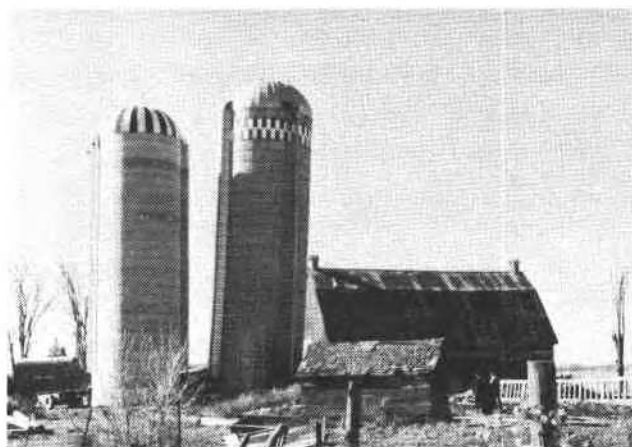
Figure 6. Foresters Falls silo, 6.10 m diameter, 21.34 m high, leaning 1213 mm from the vertical, 3 Nov. 1978.
