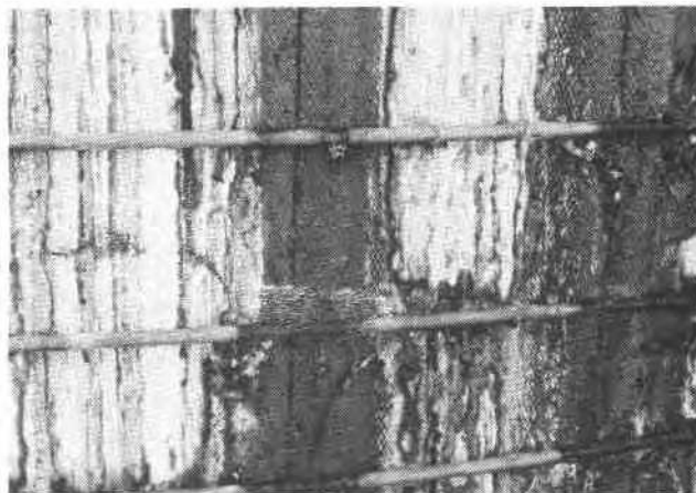
Figure 7b. Effects of structural distortion on silo: Horizontal cracks in concrete staves.
