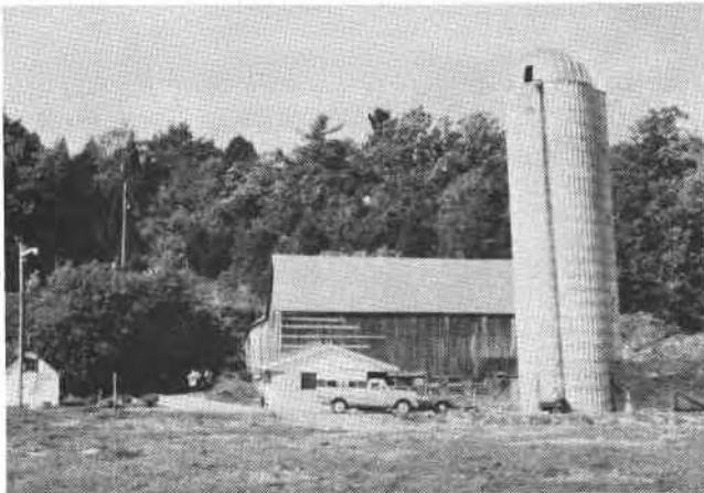
Figure 10. Mallorytown silo, 4.88 m diameter, 18.29 m high, leaning 737 mm from the vertical, 29 Sept. 1978. Rock escarpment behind barn.
